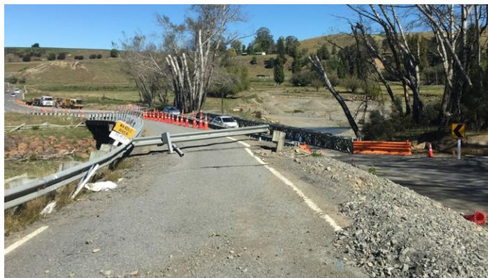
Platforms offset from the bridge have been built to enable demolition workers to sit on and munch/jackhammer the bridge from. The bridge will be 'pushed' over during a single night shift.
