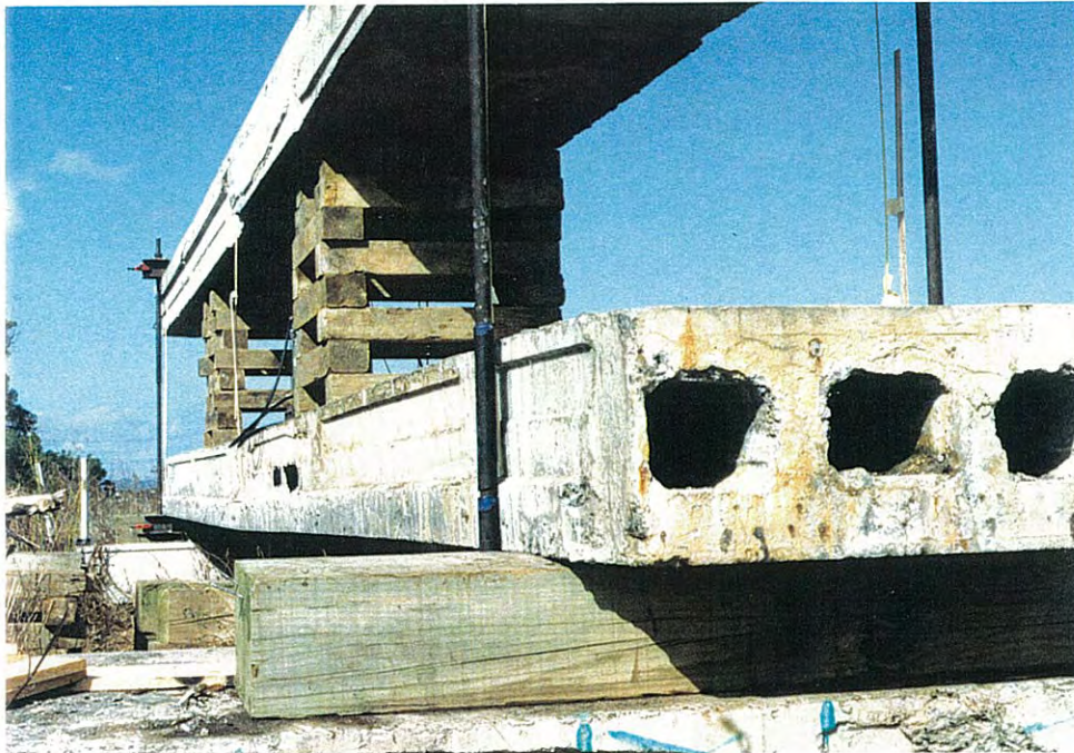
Figure 5. Test at 290 kN in first cycle. Note sag in test beam.
