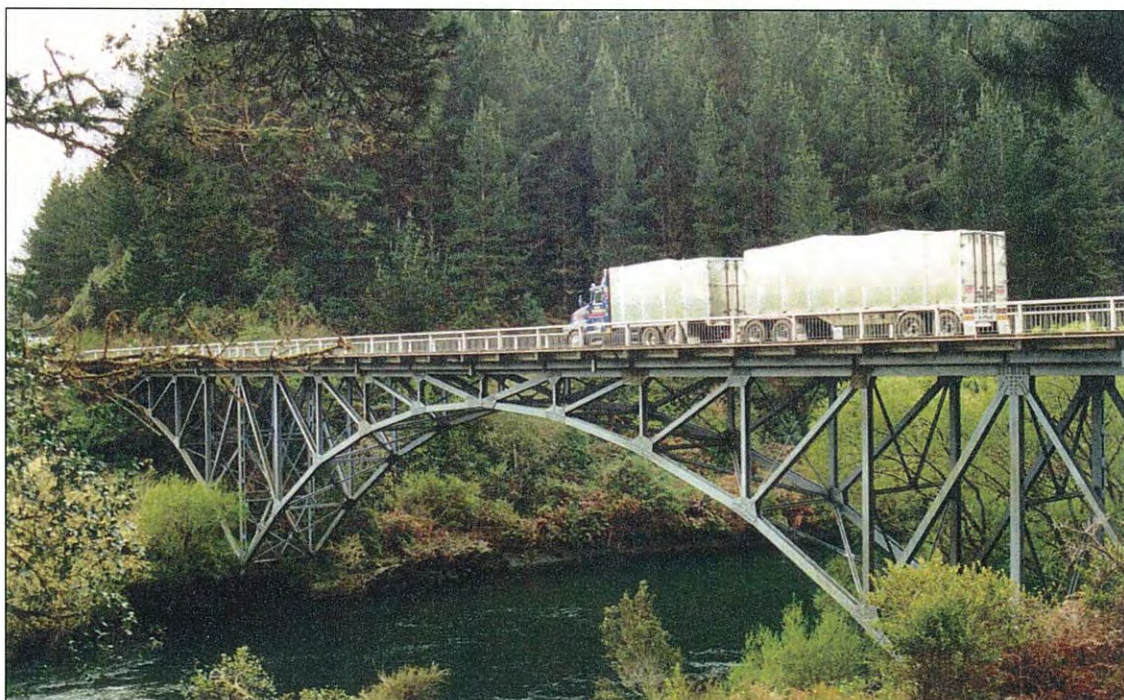
Figure 3.1 Atiamuri Bridge over the Waikato River.
