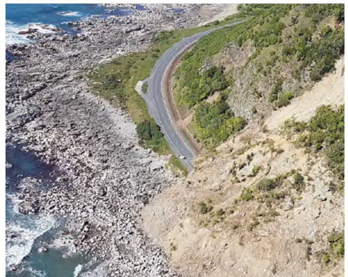
Major slip (#8) near Waipapa, north Kaikōura coast
