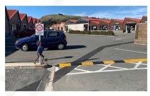
Figure 24: rubber speed hump and child crossing figure; speed limit sign non-compliant (J. Lieswyn)
