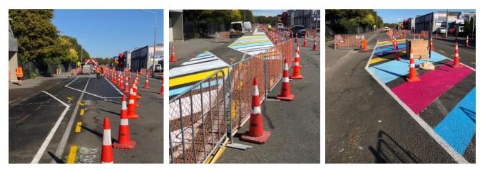
Figure 30: clean the surface, apply white primer, finish coat. Standard paint with grit mixed in is used as the surface is not going to be trafficked, Christchurch (C. Piper)
