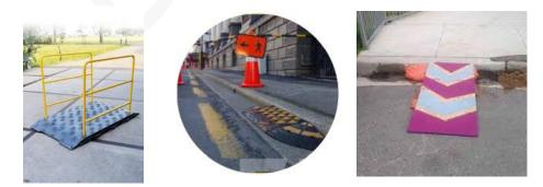
Figure 22: temporary ramps may be made of rubber, wood or asphalt (latter not pictured); must be slip resistant
