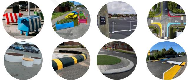
Figure 2: examples of materials used in non-permanent pilot projects
