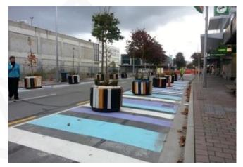
Figure 12: concrete barrel planters used for delineation, narrowing the carriageway, Christchurch (G. Dioni)
