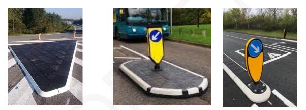
Figure 21: traffic islands made of interlocking rubber elements (left, centre) and separator kerbed islands with speed cushions (right)
