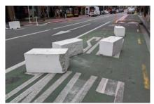
Figure 4: concrete separators dislodged, Auckland
