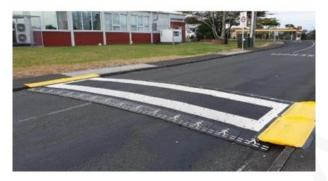
Figure 23: a platform with fillers at the kerb; markings not compliant with TCD Rule (O. McLean)
