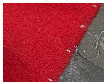
Figure 33: glue and screws used on asphalt provides for heavy skateboard and pedestrian traffic, Nelson
