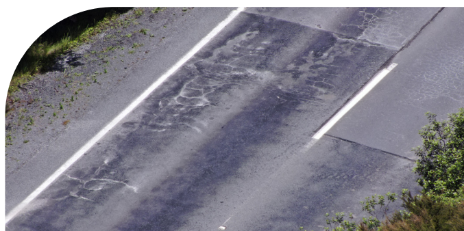
A section of SH1 Desert Road showing fatigue, cracking and rutting
