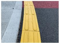
In Wellington this effect was replicated by laying yellow directional TGSI as a delineator (image at right above).
