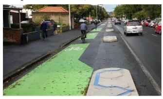
• An interesting question posed is whether to review how **cycle lanes at side roads** are marked. Some suggestions are to reduce the amount of green colouring used there (e.g. dashed blocks or lines) or to orient cycle symbols sideways to be more visible to crossing traffic. Further feedback is being sought from the AMIG team on their preferences.
