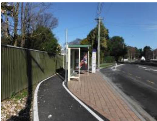
Figure 2-15: Note narrow shared use facility and restricted visibility through bus shelters
