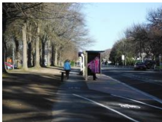
Figure 2-15: Note narrow shared use facility and restricted visibility through bus shelters
