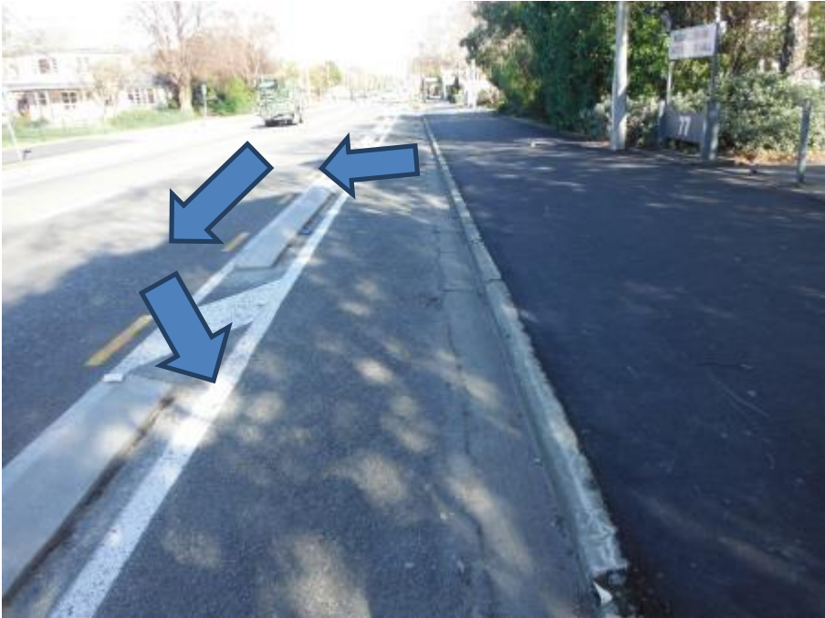
Figure 2-7 Note width of the cycle lane and the kerb restriction may make it difficult for cyclists to overtake
