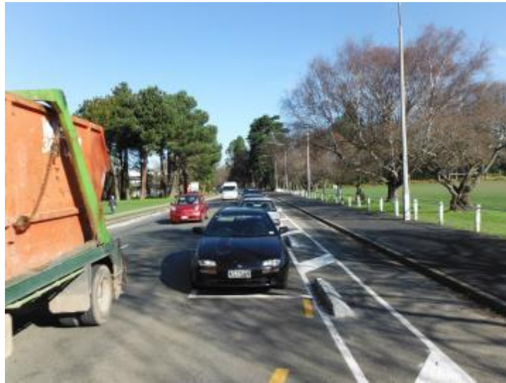
Figure 2-13: Note parking is influencing position of traffic
