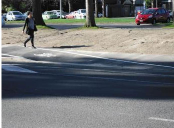
Figure 2-10: Note steep ramp on the transition to the on-road cycle lane
