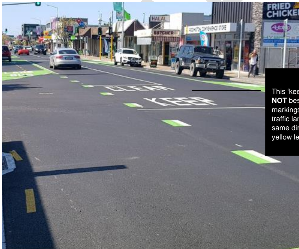
Figure 29: Keep clear marking that does not represent best practice. Source: Glen Koorey.
