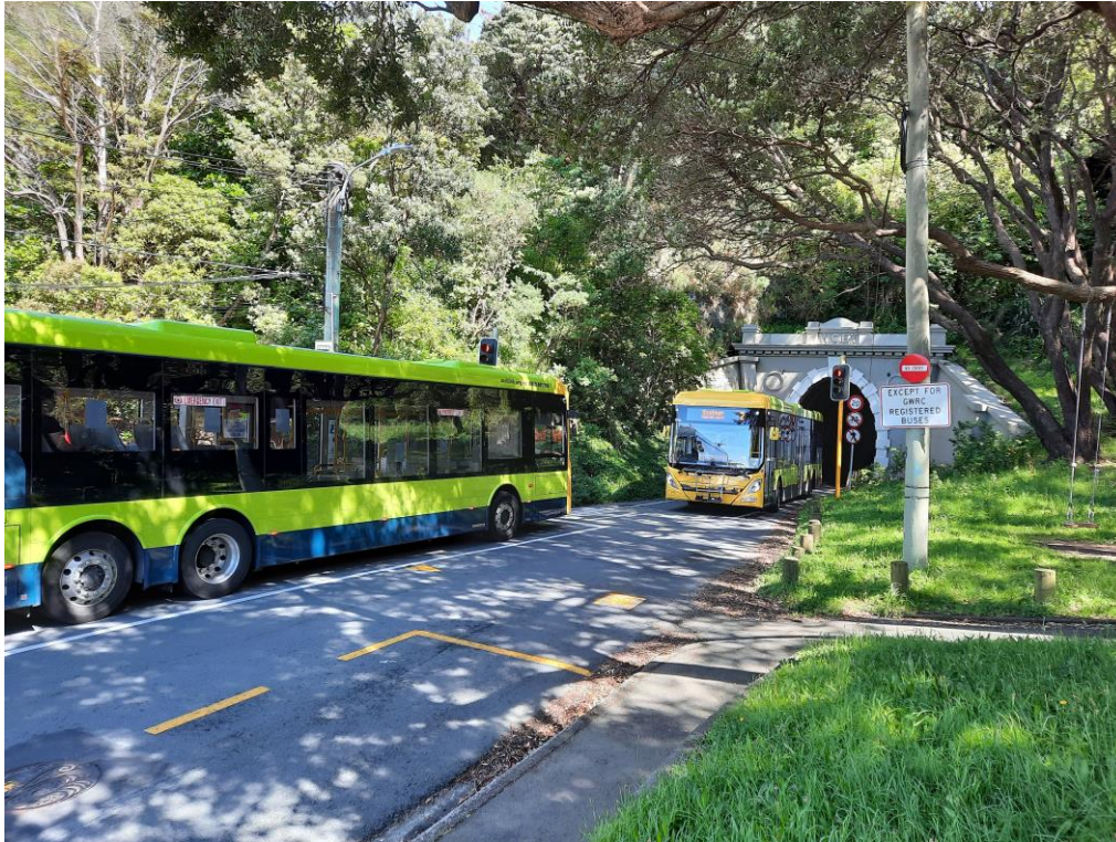
Figure 22 – One-lane, bidirectional bus tunnel with one bus waiting for another to exit the tunnel, Hataitai, Wellington. Source: Lorelei Schmitt.
