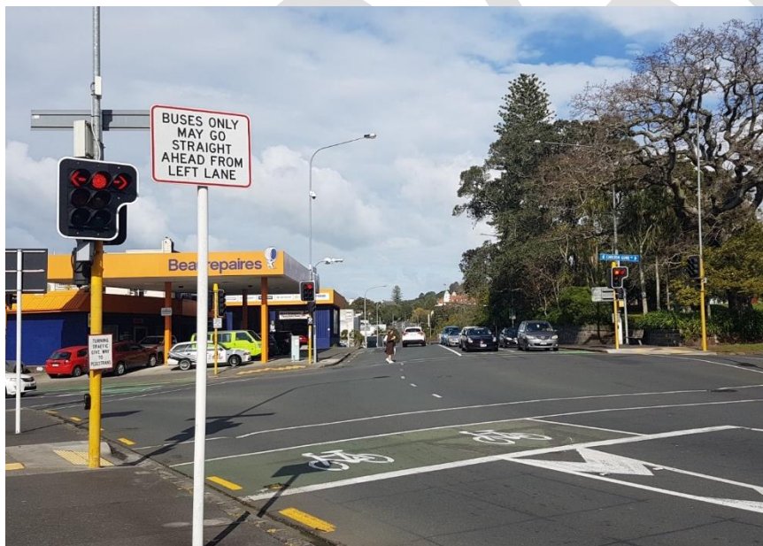
Figure 38 – Left-turn lane buses excepted facility at the intersection of Park Road and Carlton Gore Road, Auckland. Source: Aurecon.
