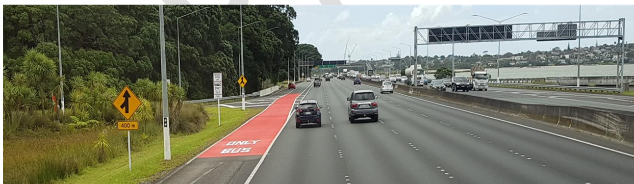
Figure 32 – Bus shoulder, State Highway 1, Onewa Road northbound on-ramp. Source: Kevan Fleckney.
