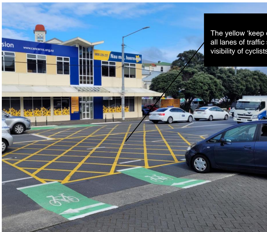
Figure 30 – Keep clear marking extending across both travel directions and the flush median. Source: Lorelei Schmitt.
