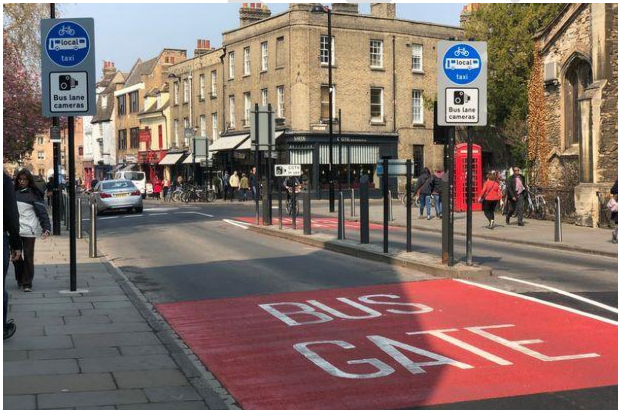
Figure 60 – Bus gate that uses enforcement cameras, Bridge Street, Cambridge, United Kingdom. Source: Cambridgeshire County Council.
