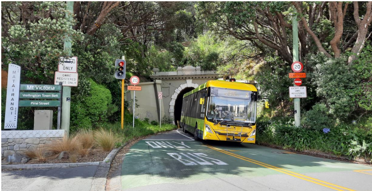
Figure 23 – B traffic signals manage the directional flows of a one-lane, bidirectional bus tunnel, Hataitai, Wellington. Source: Lorelei Schmitt.
