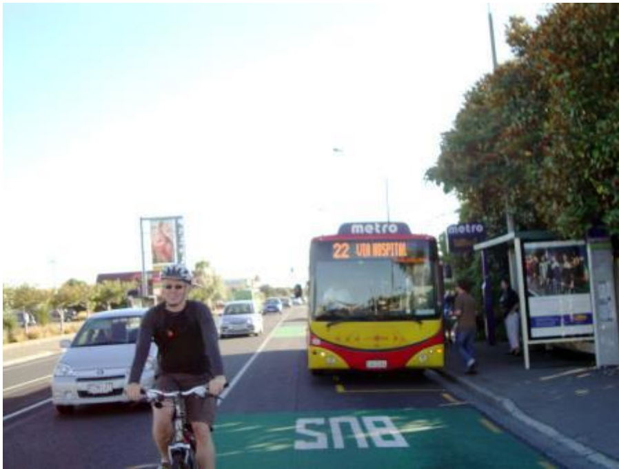
Figure 19 – Wide bus lane on Main North Road, Christchurch. Source: ViaStrada.
