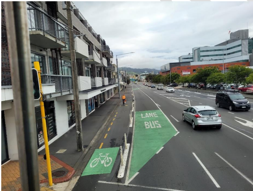
Figure 20 – Separated cycleway next to a bus lane, Riddiford Street, Wellington. Source: Lorelei Schmitt.
