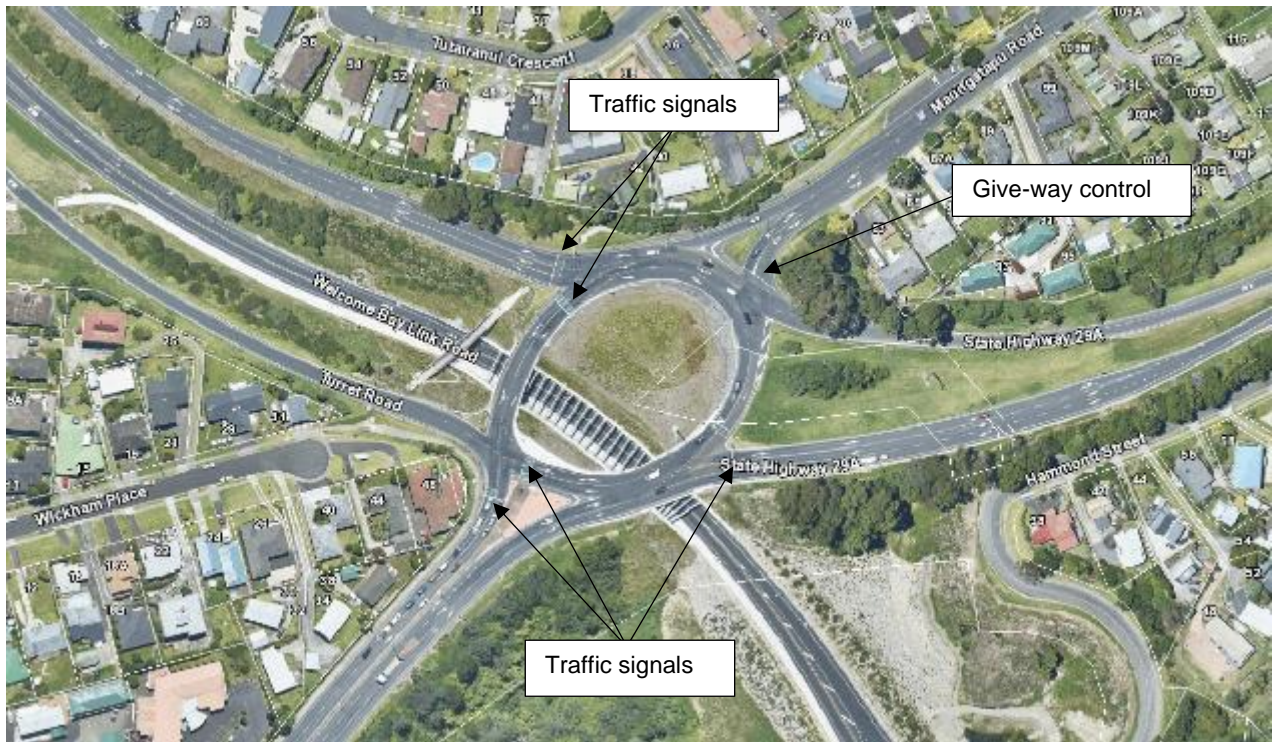
Figure 53 – Partially signalised roundabout, Tauranga. Source: Tauranga City Council.
