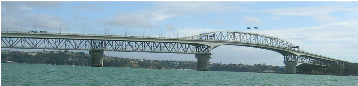
Figure 2.1. Auckland Harbour Bridge (view from Westhaven Marina)
