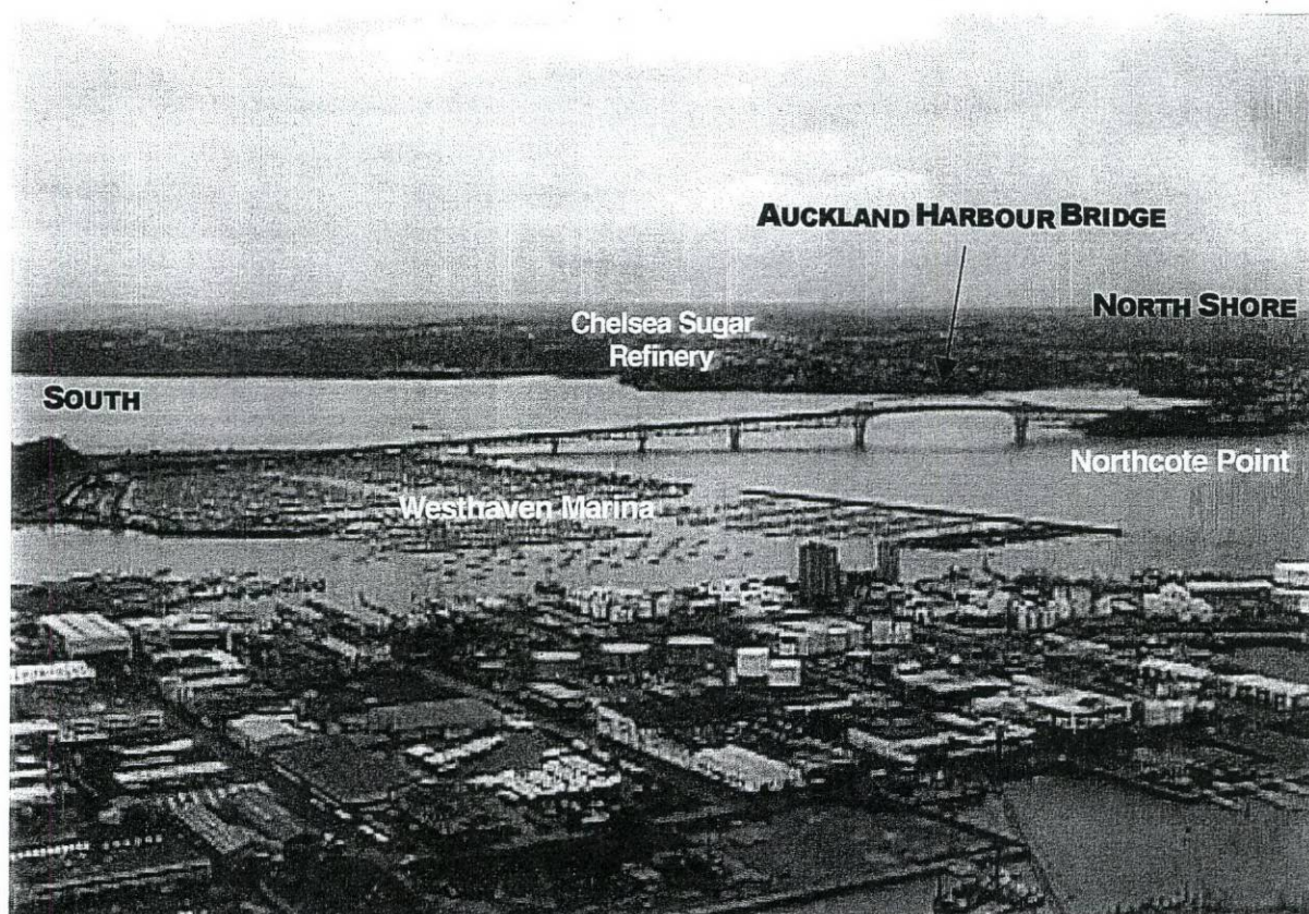
Figure 2-1 Auckland Harbour Bridge and Surrounding Area
