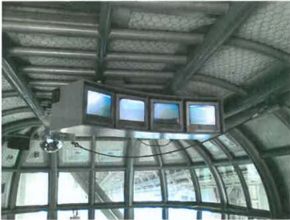
Photo 5. Sample top of screen housings TBSAJ1
