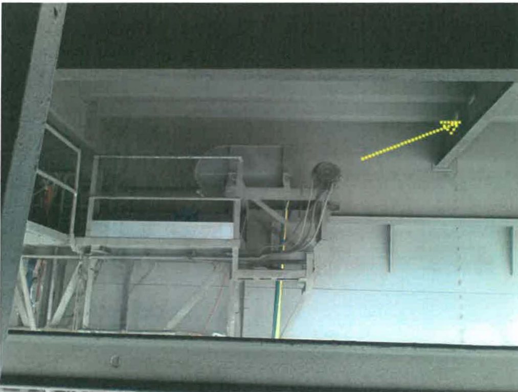
Photo 1 Area of bridge structure for abrasive blasting
