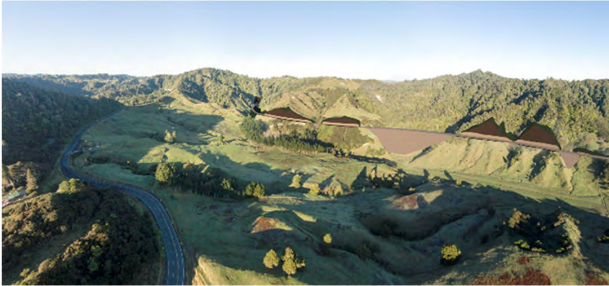
Figure 10: Option F northern approach – This approach results in landform modification along the western rural valley slopes with an alignment that cuts across the natural spur and gully pattern. This includes a large area of gully fill (mid-frame).
