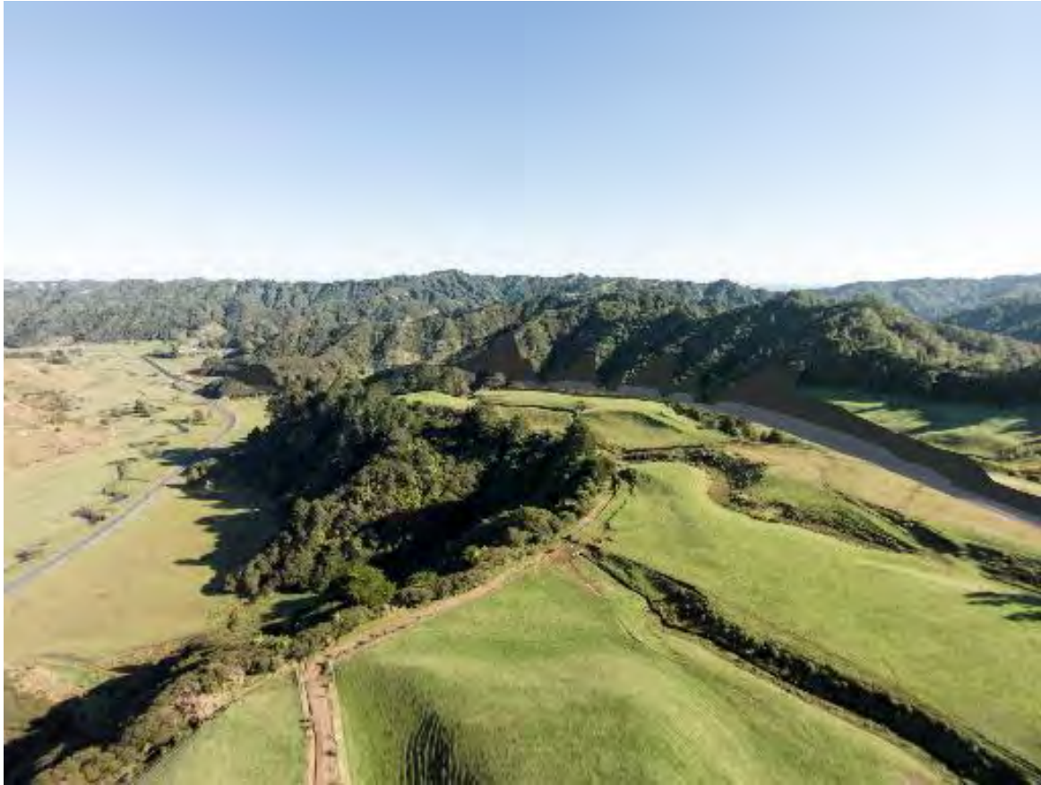
Figure 3: elevated contextual view of Option A southern approach looking south west. This image illustrates a generally cohesive orientation between highway and landform resulting in a relatively visually recessive highway section that keeps low in the landscape.
