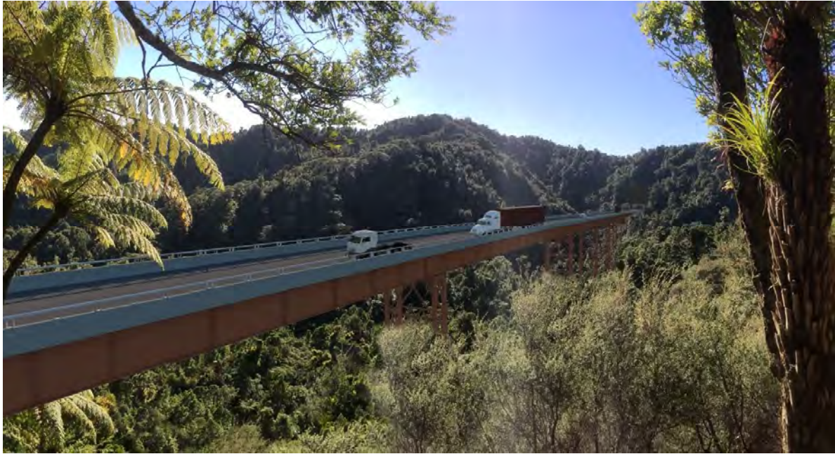
Figure 6: Option A includes a proposed 620m structure – the image above has been used to help understand the visual effects and shows a ‘baseline’ steel structure design. As discussed above this structure will introduce a significant built element into an otherwise undeveloped near pristine valley landscape. This image is also a useful guide to help understand the visual effects of possible bridge structural elements. In this image the use of steel lattice piers reduces the visual effect of vertical structures while the use of steel ‘I beams’ emphasises the visual depth of the bridges horizontal elements.
