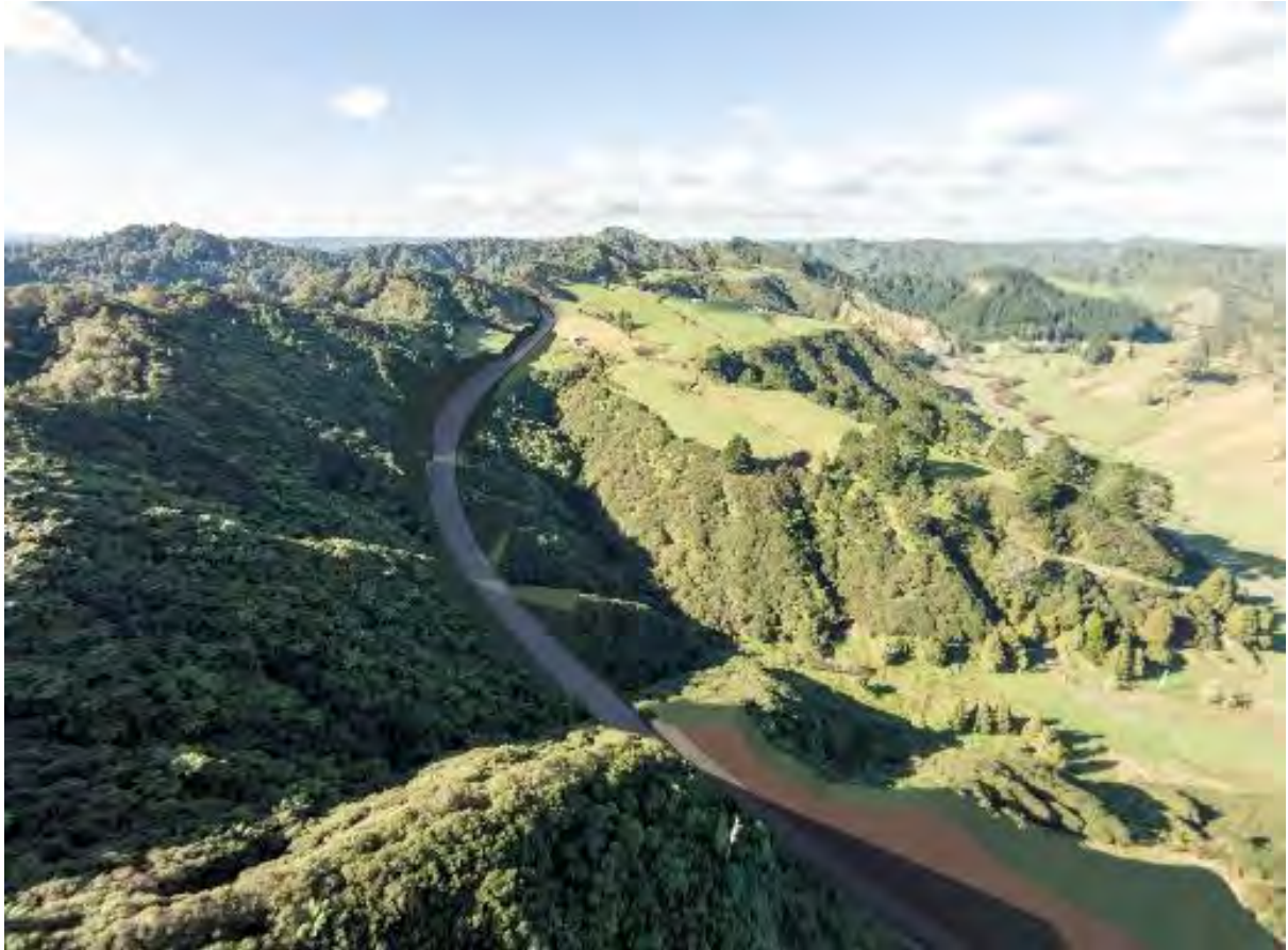
Figure 2: elevated contextual landscape view of the Option A southern approach looking to the north east. This is an improved alignment in comparison to MCA1 A options illustrating an improved highway and landform alignment.
