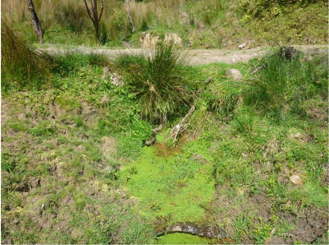
Figure C 16: Site E TL2, Mangapepeke Stream catchment, facing upstream. Cut off drain upstream draining through a 350mm culvert.
