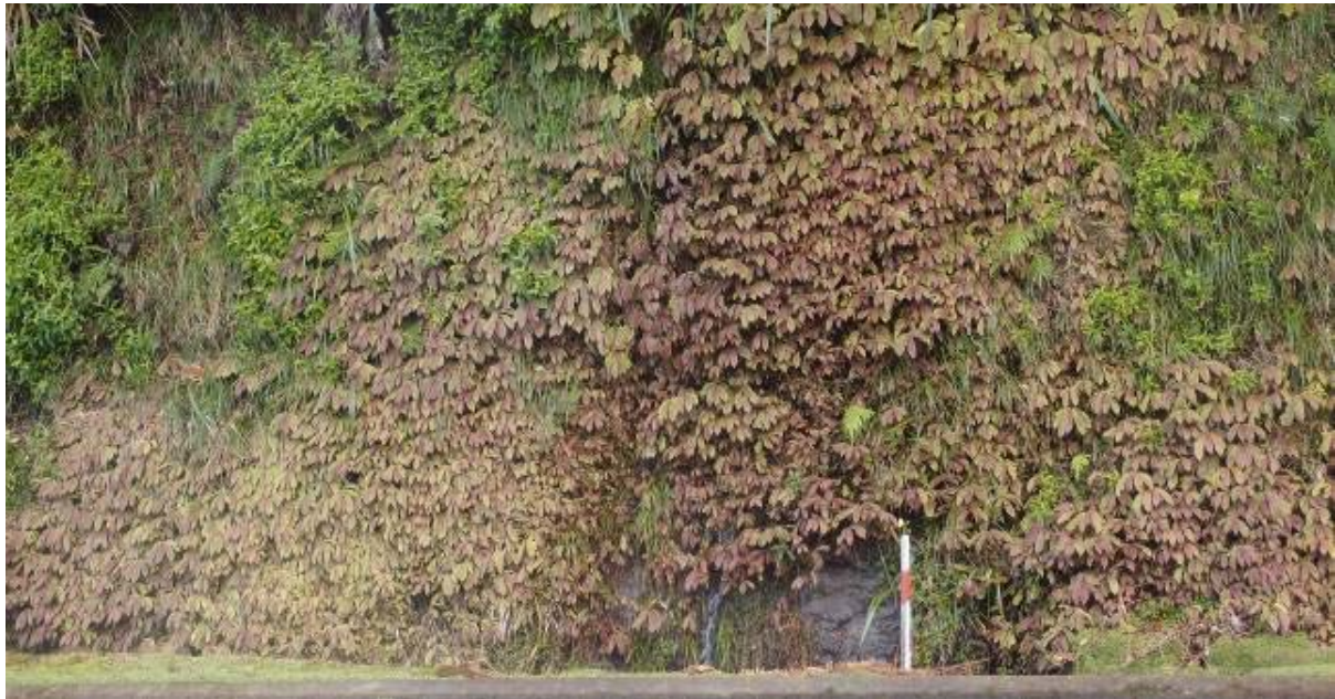
Figure 4.19 – Natural successional revegetation of existing roadside including water seepage / discharge
