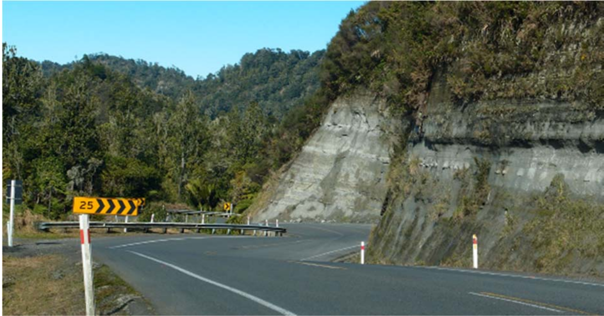
Figure 4.17 – SH3 at Mount Messenger showing the existing highway, bush hill country landscape context and naturalistic roadside character.
