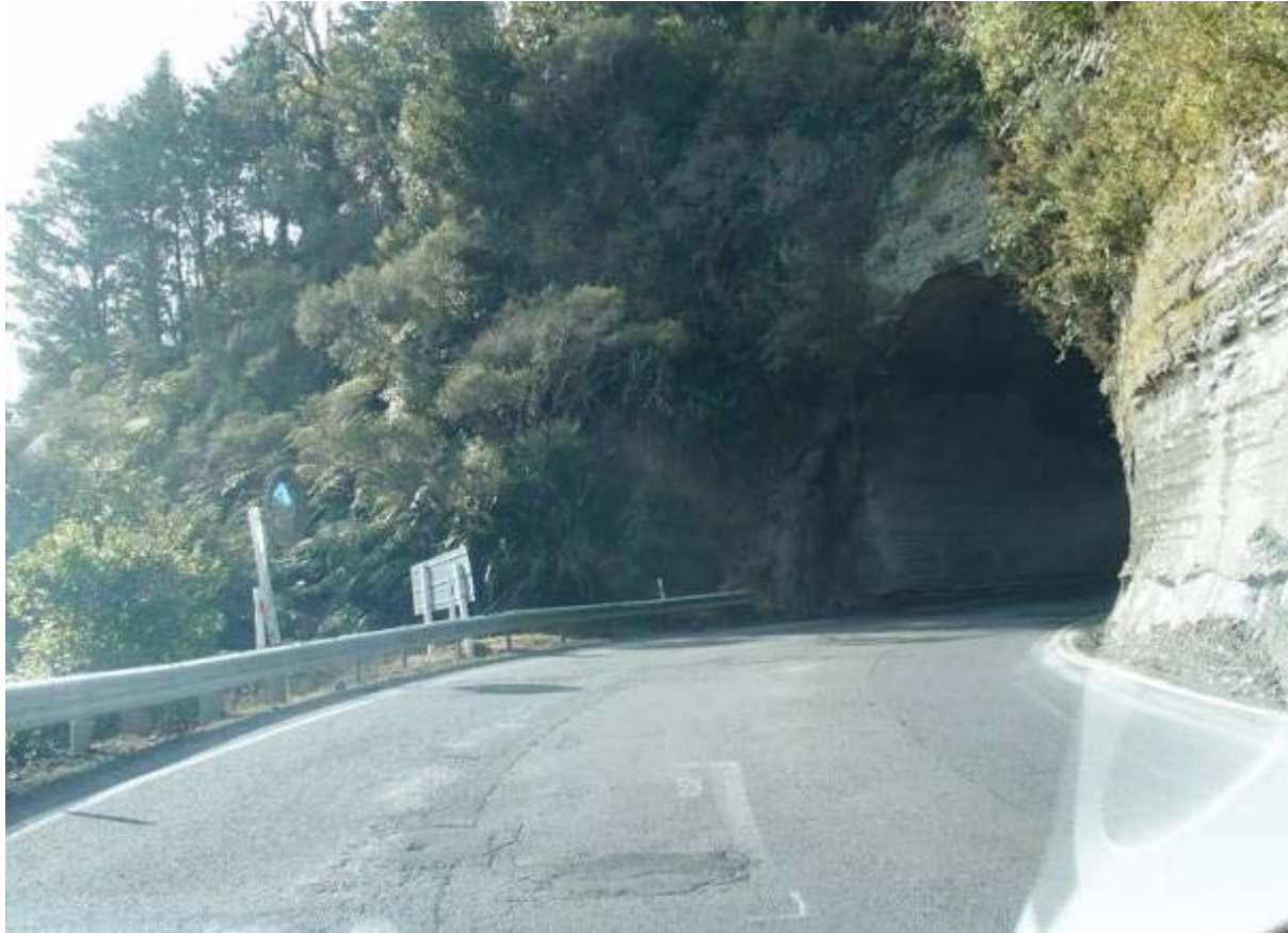
Figure 4.16 – The existing Mount Messenger Tunnel: cut directly into the papa rock, partially vegetated by natural succession.
