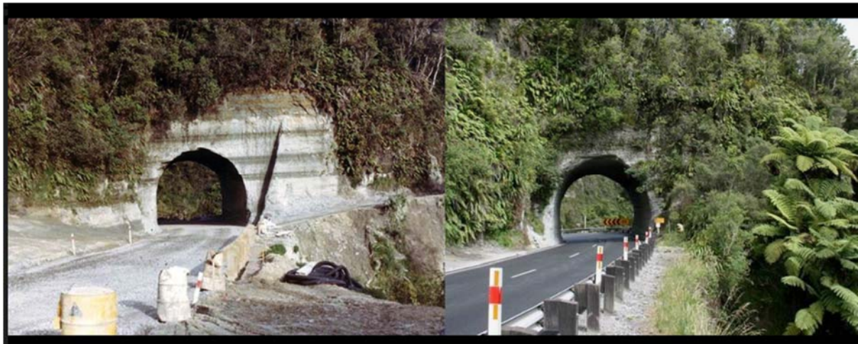
Figure 4.15 – The existing Mount Messenger Tunnel in 1983 (left) and today showing natural successional revegetation of the rock cut faces.
