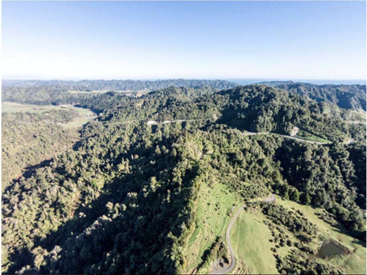
Figure 4.11 – Contextual aerial view to the south west looking towards Mt Messenger (centre frame) and the Mimi Valley (left of frame). Pastoral flats can be seen left of frame defined in part by SH3 and the Mimi Stream. The existing SH3 roadway can also be seen in this image as it winds its way across the Mt Messenger landscape.
