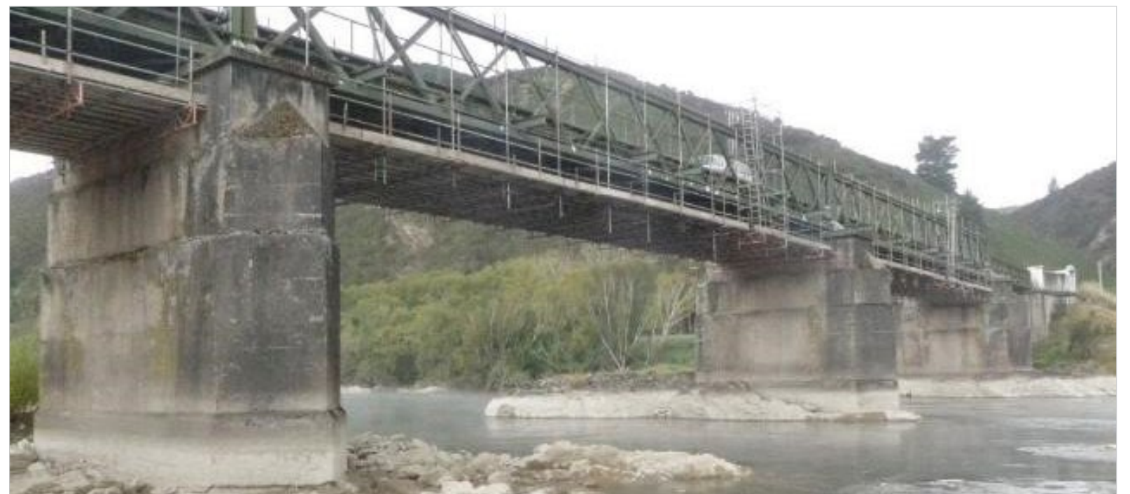
b) Elevation of existing bridge showing buttressing to piers and geometry of wrought iron trusses FIGURE 8: EXISTING BRIDGE PHOTOS
