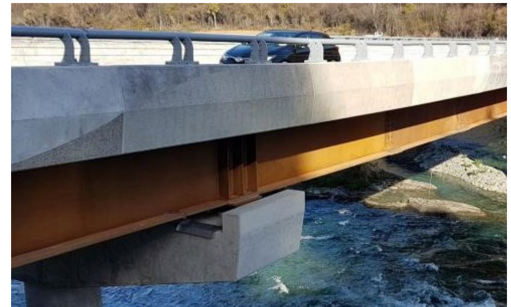
FIGURE 15: EXAMPLE OF WEATHERING STEEL USED FOR BRIDGE GIRDERS AT KAWARAU FALLS BRIDGE NEAR QUEENSTOWN. THE KAWARAU FALLS BRIDGE ALSO INCORPORATES TEXTURES IN THE OUTSIDE FACE OF “HT” CONCRETE BARRIERS.
