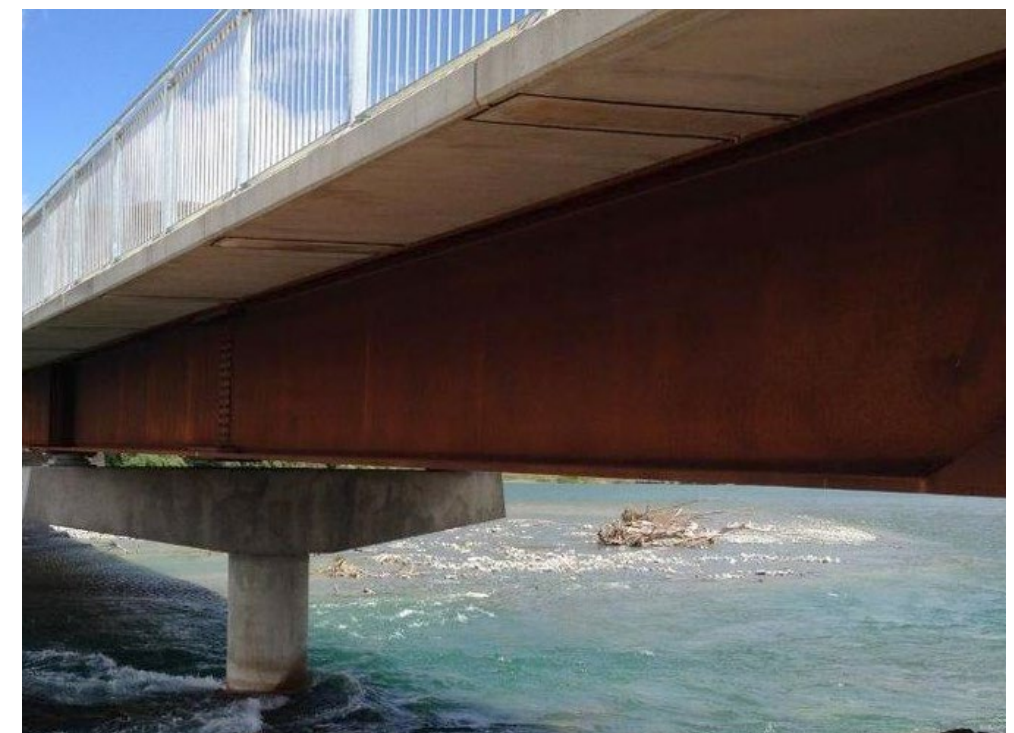
FIGURE 16: EXAMPLE OF WEATHERING STEEL USED FOR BRIDGE GIRDERS ON THE WAITAKI RIVER BRIDGE, KUROW.
