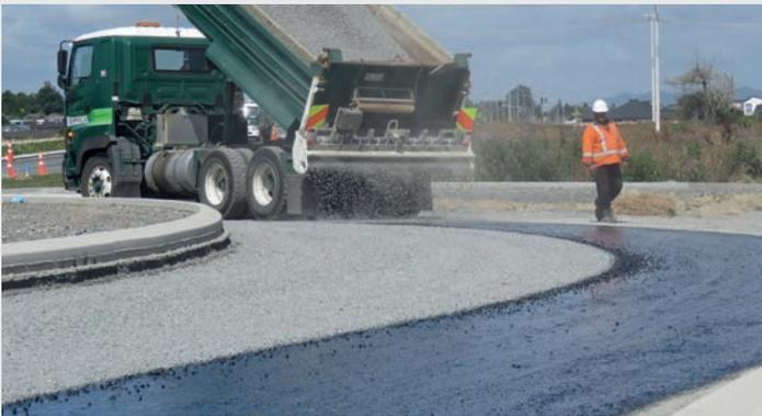
The road is sealed with stone chip, then asphalt.
