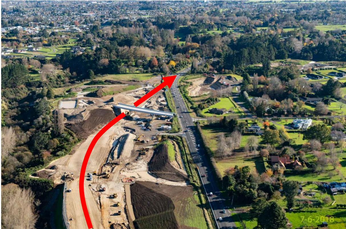
We're building two new lanes to run from the Airport Road Interchange, under the East West Link Bridge, reconnecting with SH1 at the top of the gully near the 'Hamilton' billboard. The red line shows where these lanes are being constructed. The new lanes will be sealed in October/November and SH1 traffic switched on to these lanes. The old highway will be closed north of Cherry Lane.
