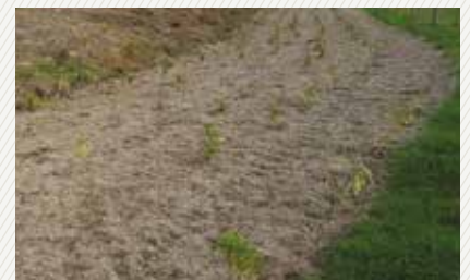
Planting is already under way.
