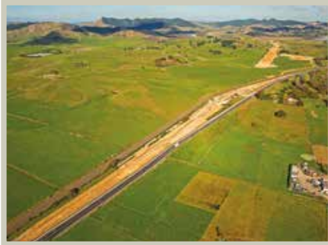
Huntly Northern Interchange
