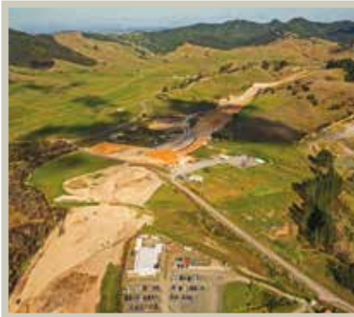
Works to the south of McVie Road
