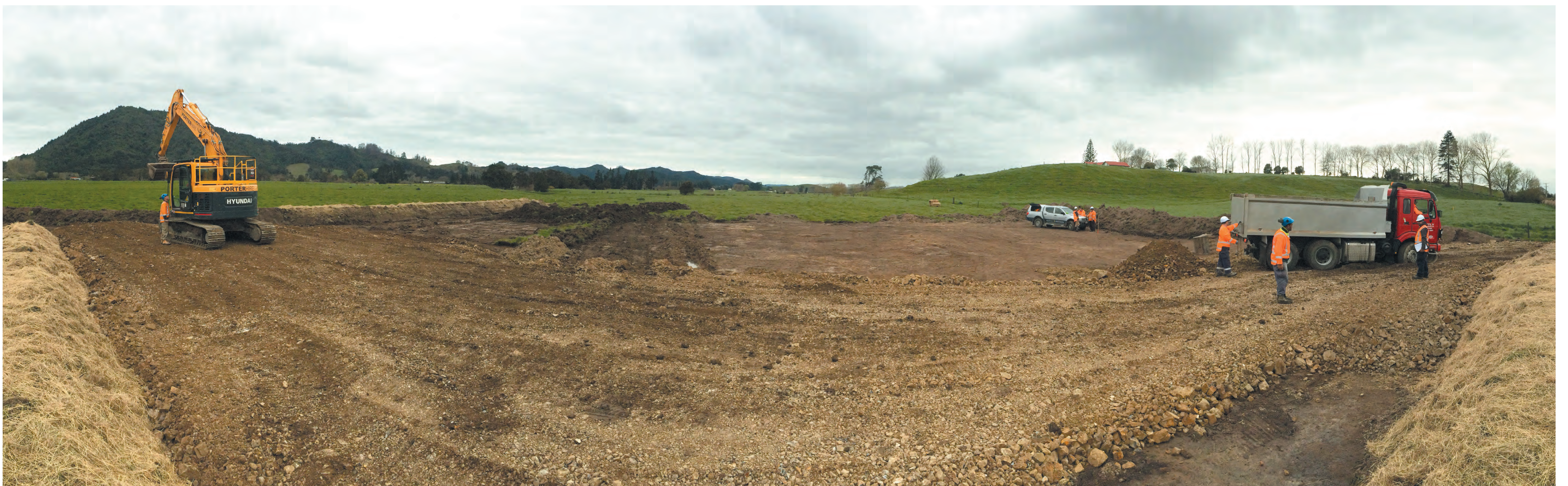
Site works at Waring Road
