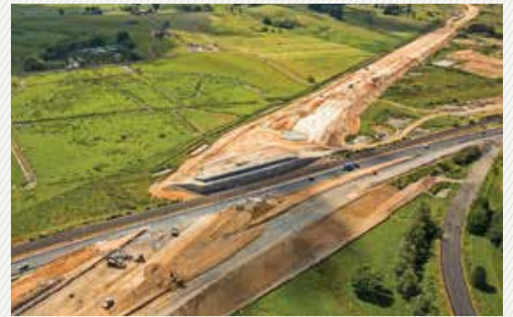
An aerial view showing progress on the Northern interchange
