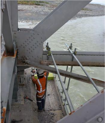
The next crew start at 2pm to core 1m deep bore holes for the replacement bearings anchor bolts. The removal team returns, becoming the installation team from 1am.
