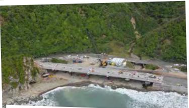
Irongate Bridge, the fastest seven-span bridge build in New Zealand. The bridge has been moved across the rail line, closer to the coastline. There is a new seawall to the north which the bridge lands on, and a slightly reshaped rocky bluff to the south. This has allowed for a straighter, safer road alignment.
