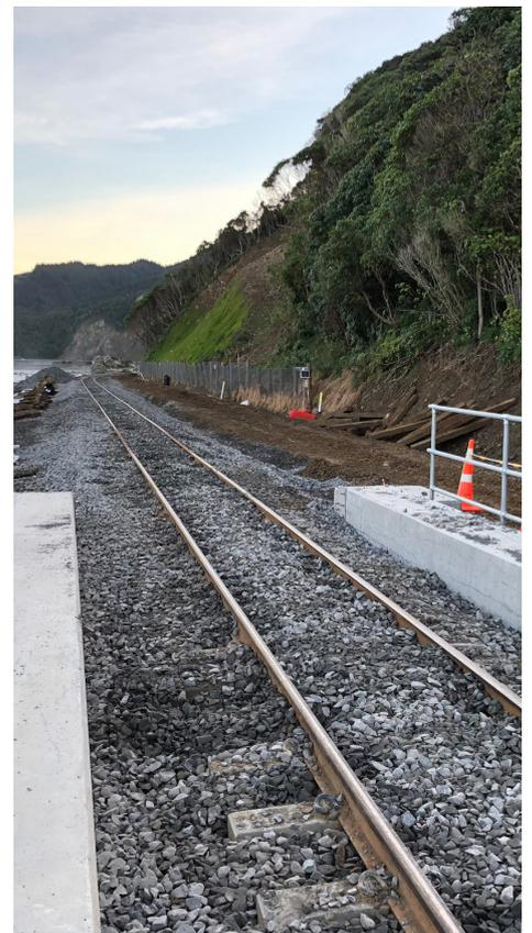
A KiwiRail team has placed railway track onto the third and final debris-flow rail bridge between Half Moon Bay and Ōhau Point, north of Kaikōura. A channel is now being dug under the bridge, which will allow material from the hillside above to pass underneath. After those earthworks are complete, the next step is concreting the channel.
