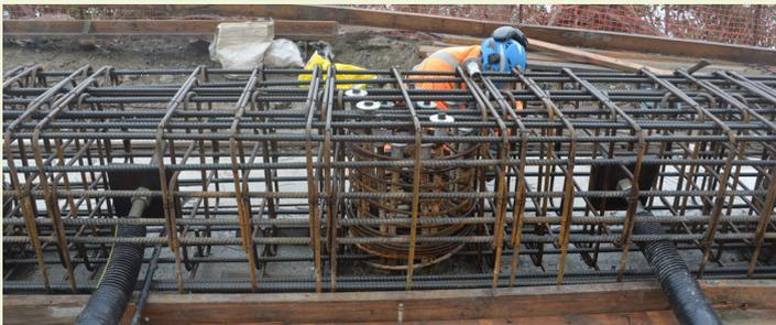
48 reinforced concrete piles were constructed to a depth of 13-22 metres. The concrete at the top of each pier is removed to expose the steel reinforcing rods. These rods, as well as the rock anchor ends, are then tied securely into a complex steel reinforcing cage that will form the skeleton inside the capping beam.
