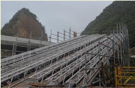
Rock anchors consist of a steel rod grouted inside a plastic tube. This ramp allows grout to be poured into the tubes at the correct 15 degree angle, to secure the rods at the same angle they will go into bank.
