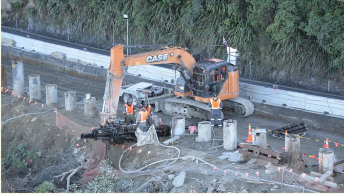
Pre-drilling 18-metre rock anchor holes under the road, and into the rock bank, at angles of 15 and 30 degrees. A fine mist is sprayed to reduce dust.
