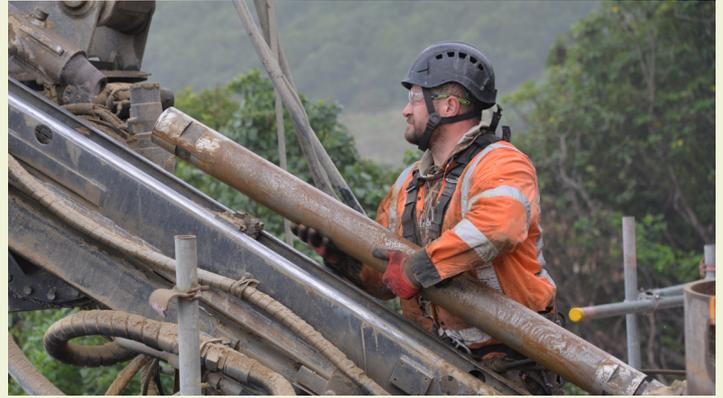
Supervisor Lukis Fuller adding a length of casing to the rock drill.
