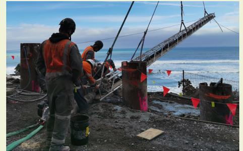
Pre-grouted rock anchors are swung into position by crane, then inserted into the pre-drilled holes.
