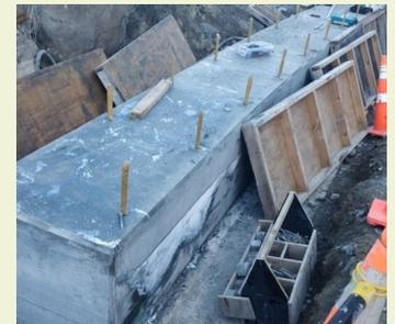
The concrete is poured in multiple sections, with a gap between each segment to allow for earth movement. Once complete, the road can be built up to finished level, and guardrails installed. Road sealing should take place in October, once weather conditions are suitable.
