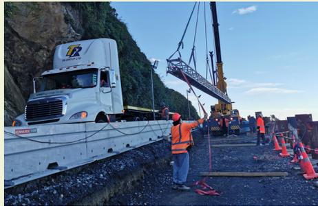
Before work started, a platform was built to hold the machinery, and a crane sourced that would fit the narrow corridor, but is large enough to manoeuvre a rock anchor around into the hillside.
