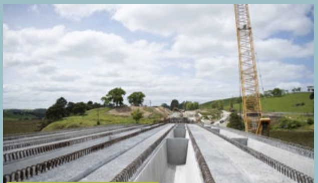
Looking eastwards across Bridge No.2 super tee beams
