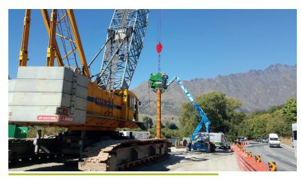
The 150 tonne Crawler crane that will drive the piles for the trestles that will extend out into the river, to provide a platform for workers to build the new bridge piers.
