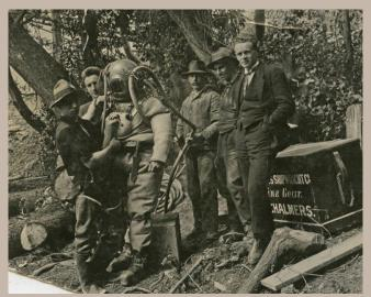
Times have changed but the crew at the new Kawarau Falls Bridge project still use divers for important close underwater construction work. Most of the time, the team uses a Go Pro strapped to some scaffolding, which is lowered down into the river to carry out underwater inspections. This difficult, dangerous and time consuming work previously carried out by people in diving suits is now done by cameras both quickly and safely.
