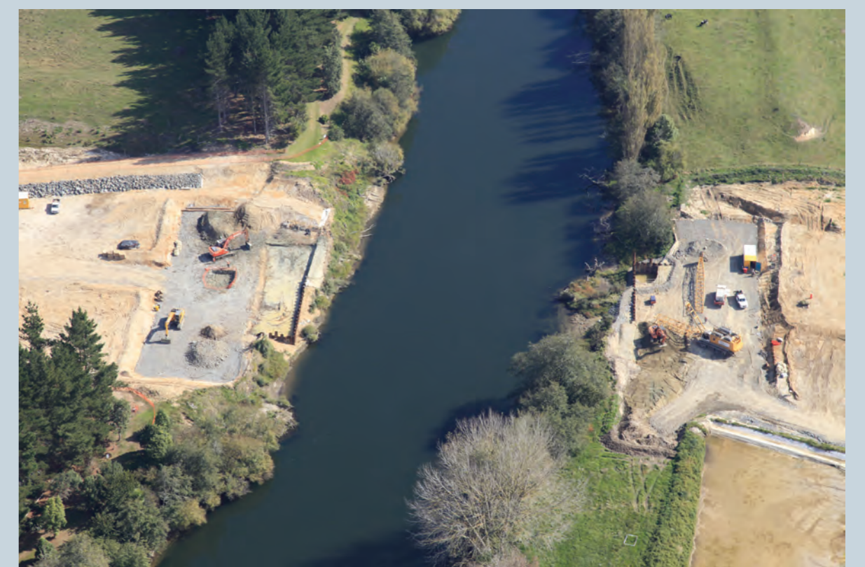
Waikato River Bridge construction, April 2012
