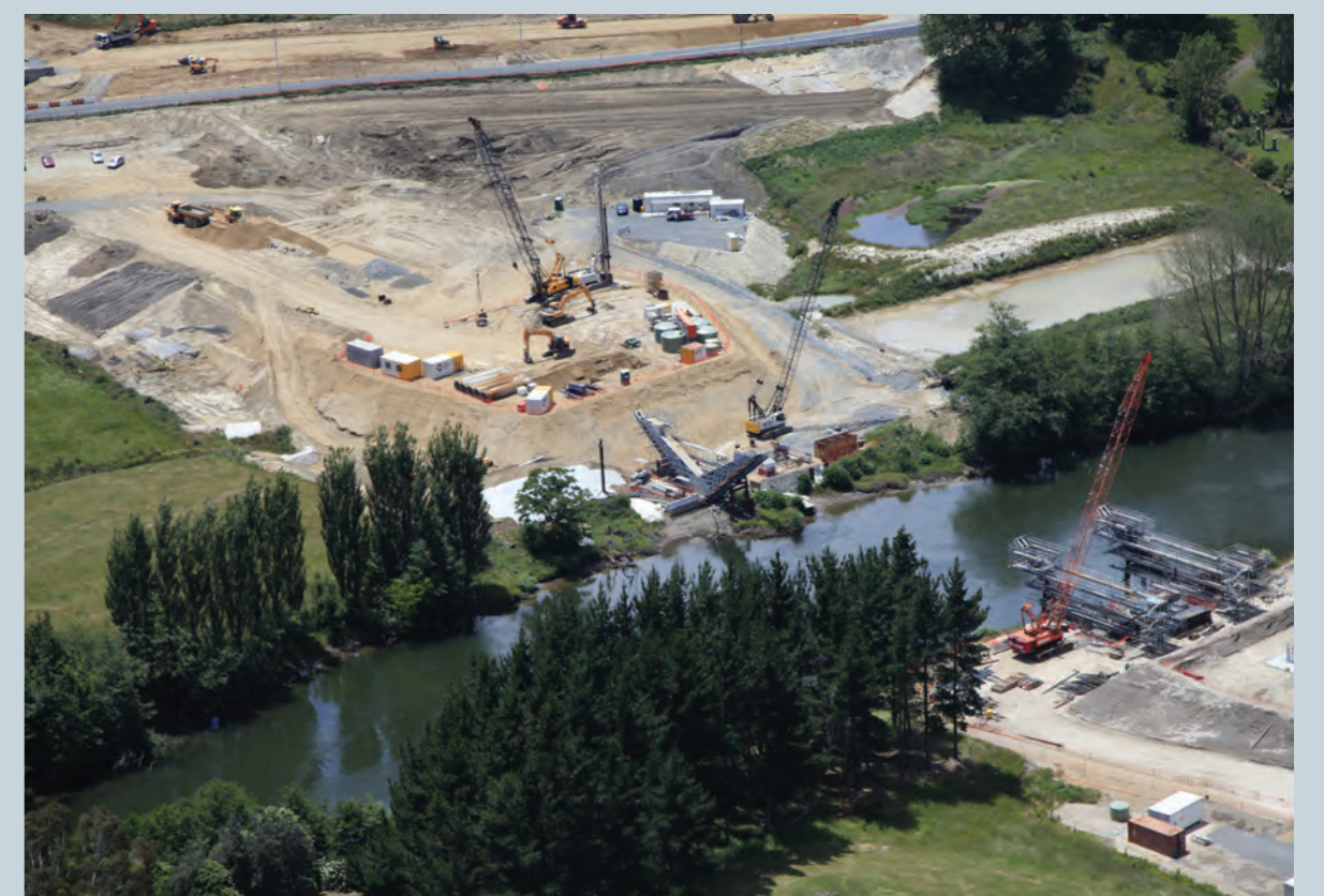
Waikato River Bridge pier construction
