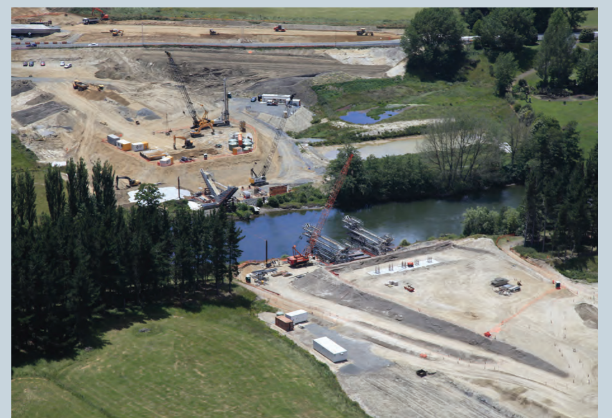
Waikato River Bridge pier construction
