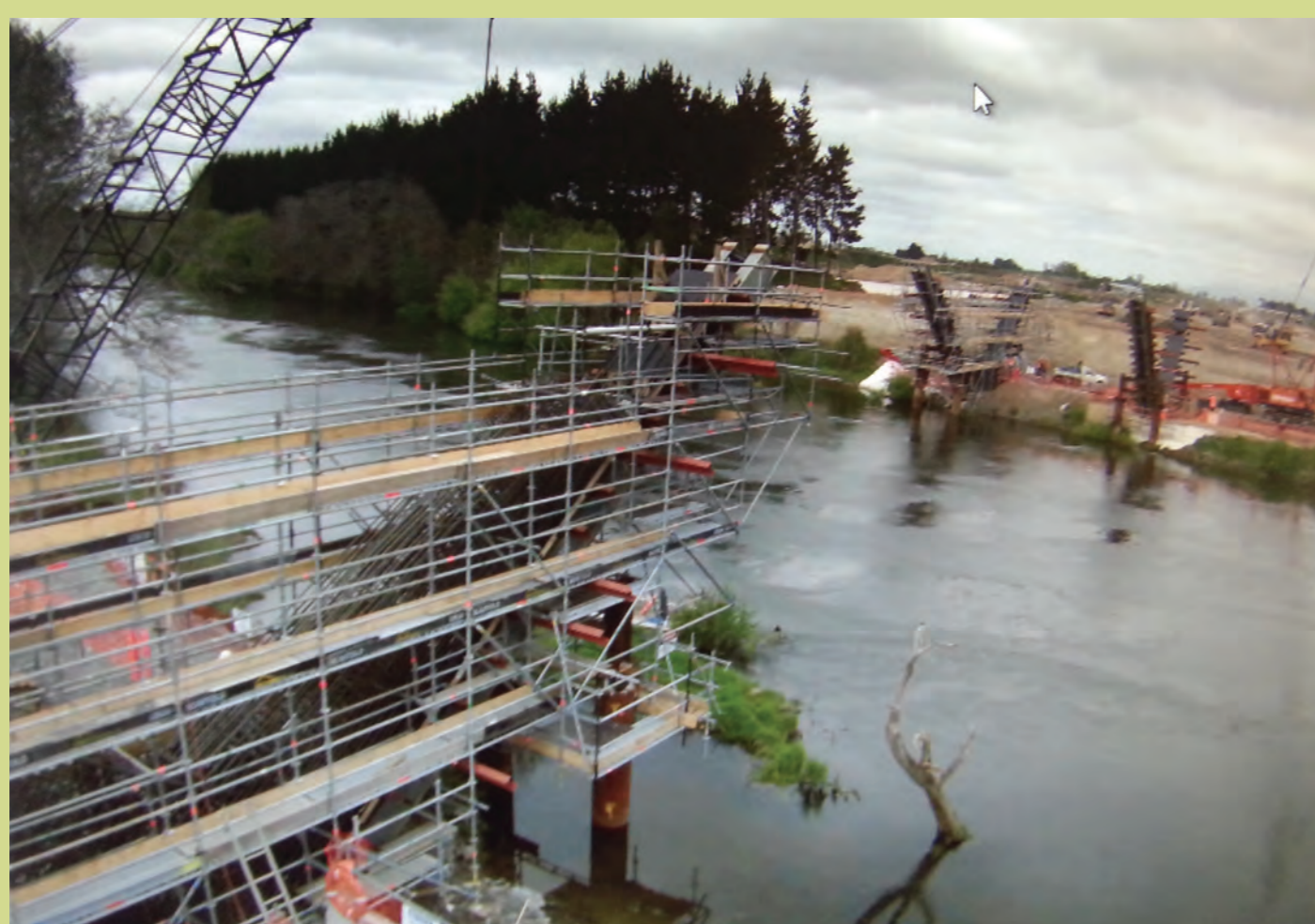
Bridge 'V' piers under construction, October 2012
