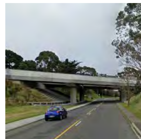
Highway over local road [Google Street View]
