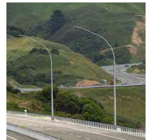
Highway light pole example, Te Ara Nui o Te Rangihaeata, Transmission Gully [Waka Kotahi]
