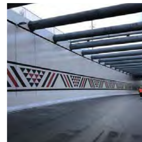
Maungatapu underpass [ https://www.nzta.govt.nz/media-releases/maungatapu-underpass-artwork-revealed/ ]
