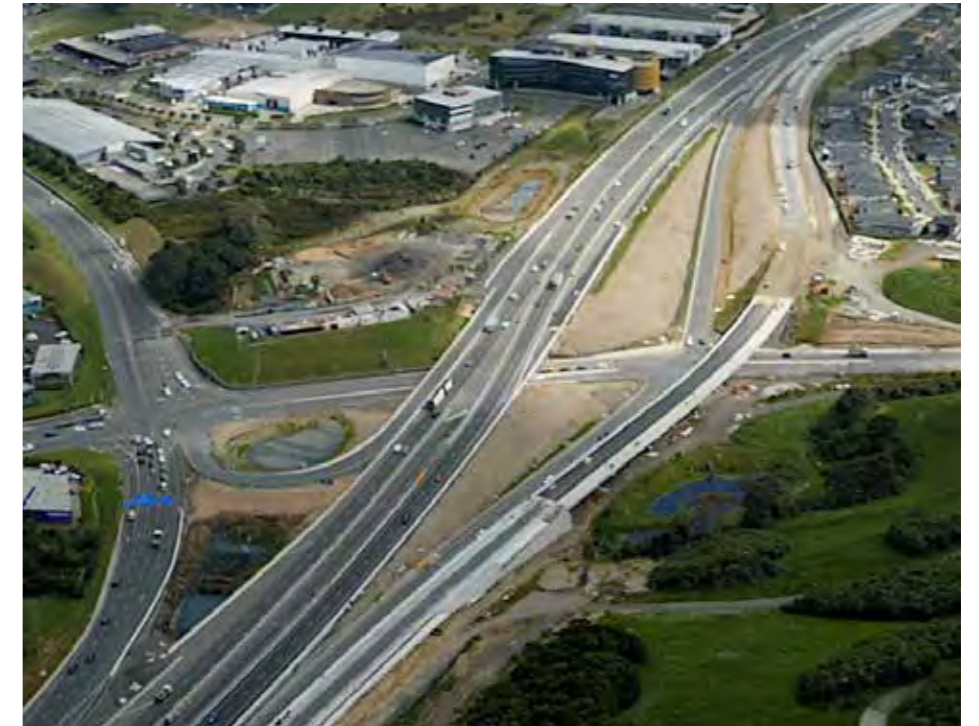
Top: Northern Corridor Improvements Illustration of integration of earthworks into surrounding [Waka Kotahi] Below: Mackays to Peka Peka expressway [ https://www.naturalhabitats.co.nz/our-projects/mackays-to-peka-peka/ ]
