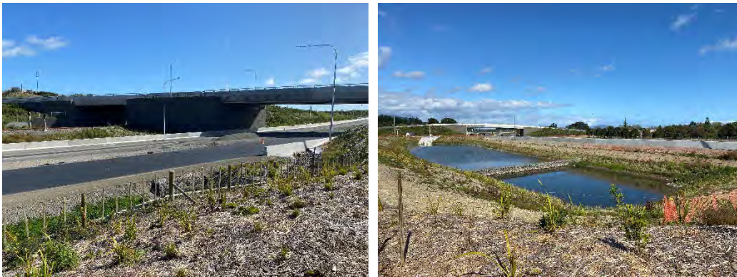
Figure 10 New State Highway being completed south of Ōtaki
