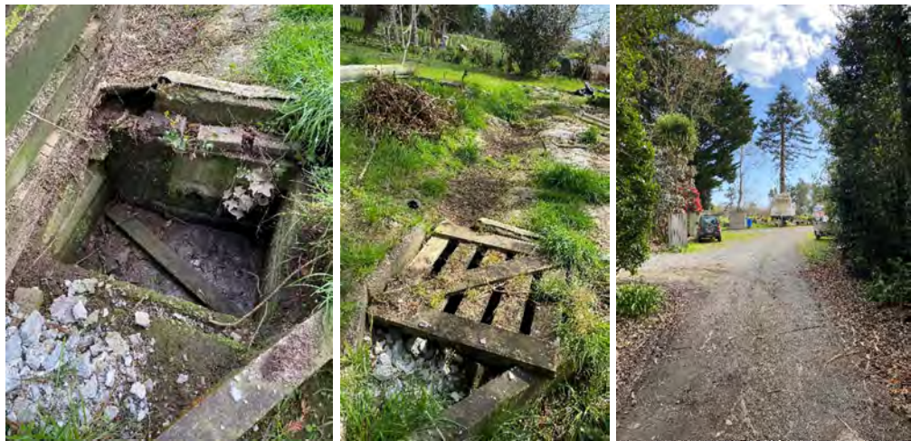
Figure I.3 Sump and soak away area at 380-386 Arapaepae Road (HAIL ID 10)
