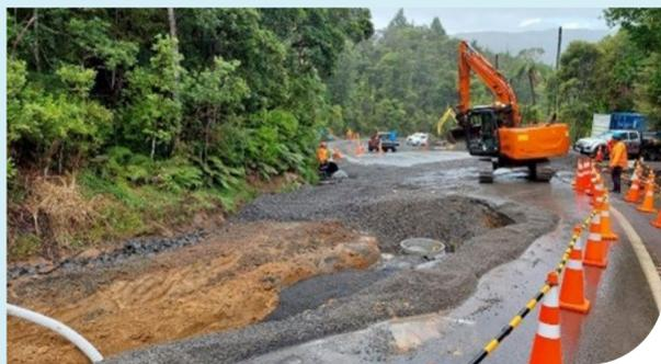
Effective stormwater and sediment management plays a major role in protecting the environment through construction. We're installing silt fencing, rainwater capture drains and sediment tanks to ensure any stormwater runoff is collected, diverted, and treated before it reaches the local waterways.
