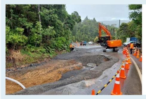
Effective stormwater and sediment management plays a major role in protecting the environment through construction. We're installing silt fencing, rainwater capture drains and sediment tanks to ensure any stormwater runoff is collected, diverted, and treated before it reaches the local waterways.
