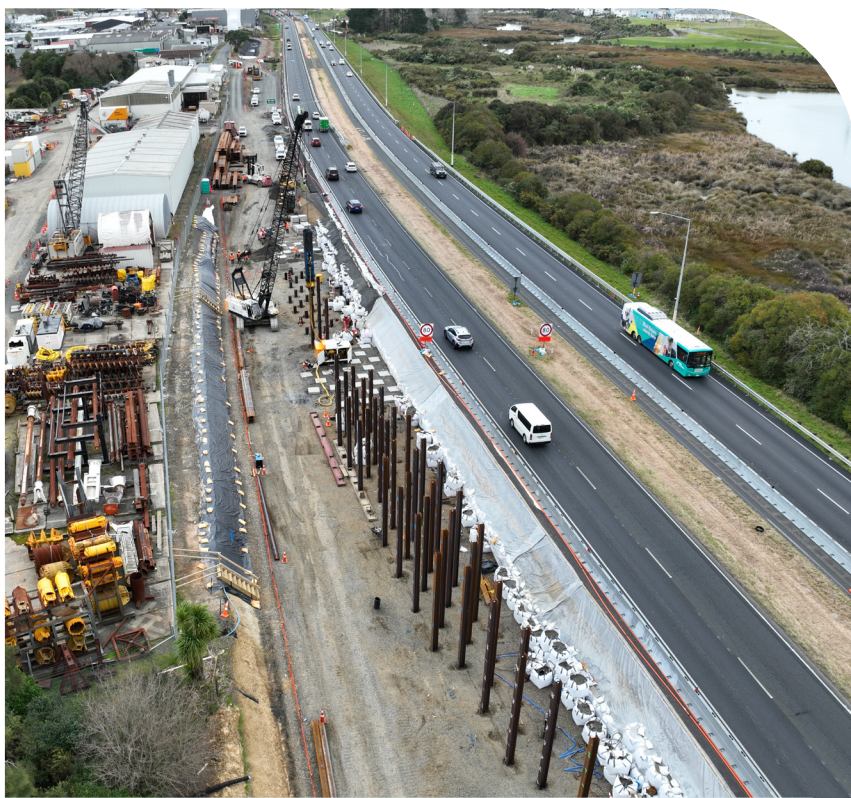
Driving UC piles to strengthen the ground south of Slippy Creek/Otuuwaioa Stream.
