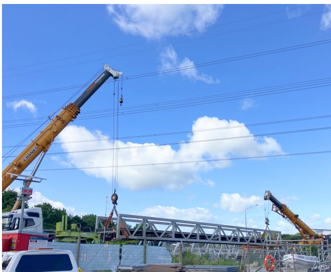
Both spans were lifted out using 170 and 130 tonne cranes.
