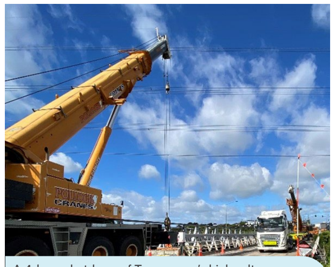
A 4-hour shutdown of Transpower's high voltage power lines directly above the pedestrian bridge was required for this lift.
