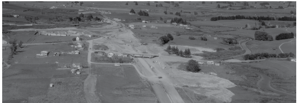
Near Drury Interchange in September 1965, with construction already underway on the motorway extension and the Bremner Road bridge. The Takaanini to Drury section of the motorway officially opened in December 1965, and Drury Interchange was completed in 1967.
