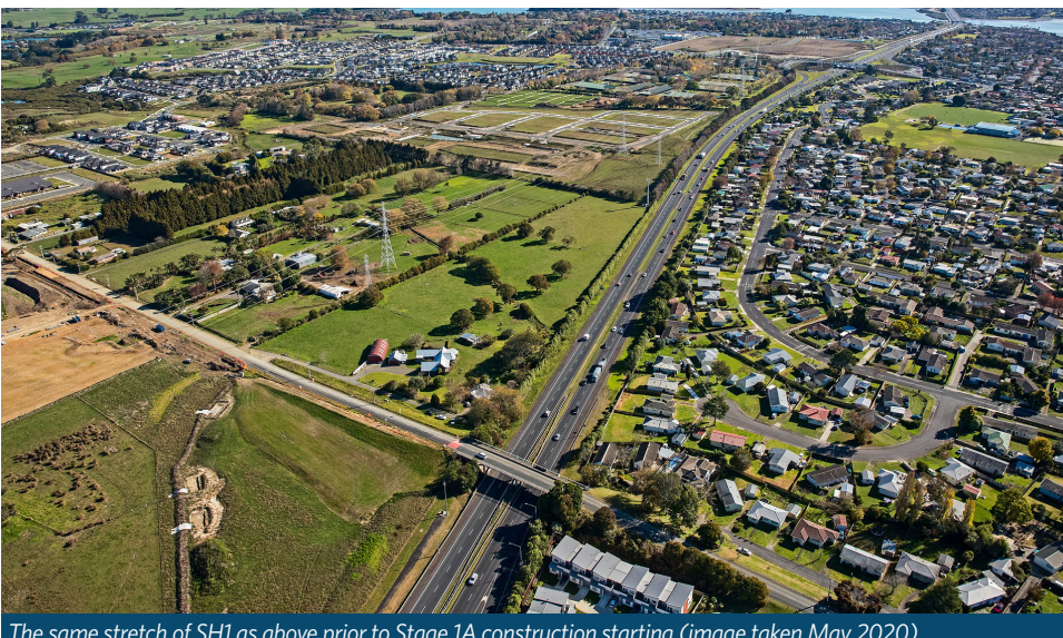
The same stretch of SH1 as above prior to Stage 1A construction starting (image taken May 2020).
