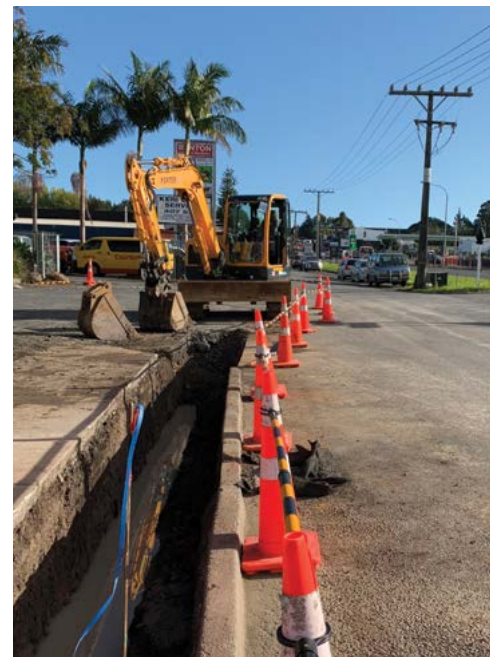
Digging a shared service trench on Skippers Lane
