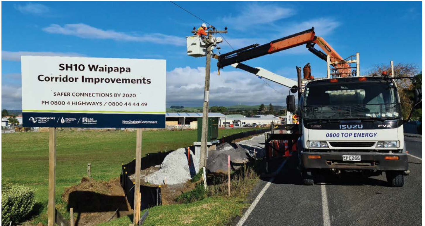
Moving power cables underground on Waipapa Road
