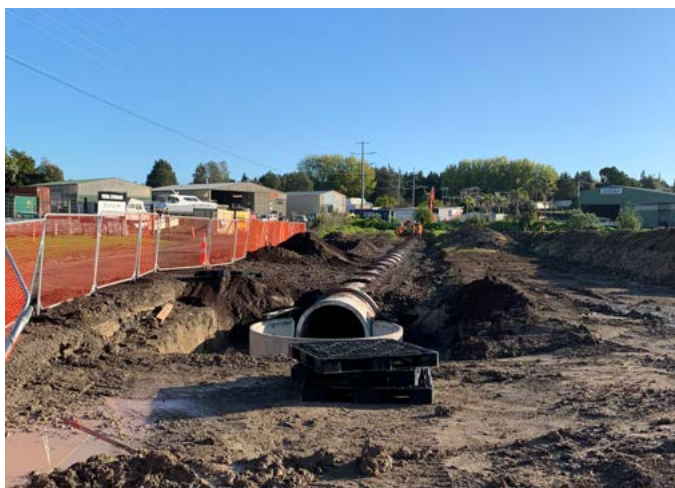
New stormwater pipes on the site of the Maritime Lane extension
