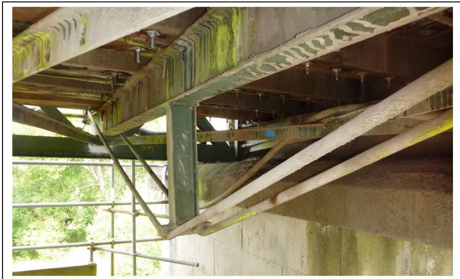
King Post/Tie Rod Transom Strengthening
