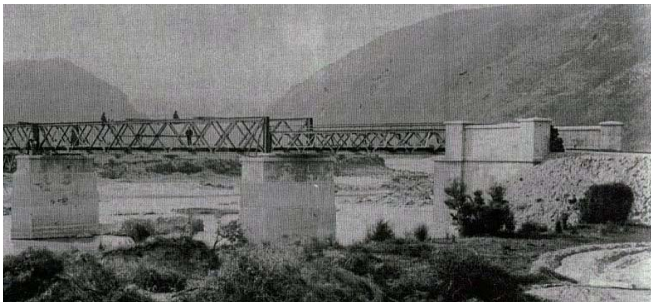
Figure 23: Beaumont Bridge in 1887, thought to be around the time of its opening.
