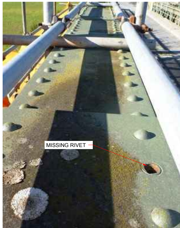
A RIVET IS MISSING ON THE TOP OF THE TOP CHORD, A M20 BOLT SHALL BE INSTALLED TO REPLACE THE MISSING RIVET. TOTAL PLATE THICKNESS IS 51mm
