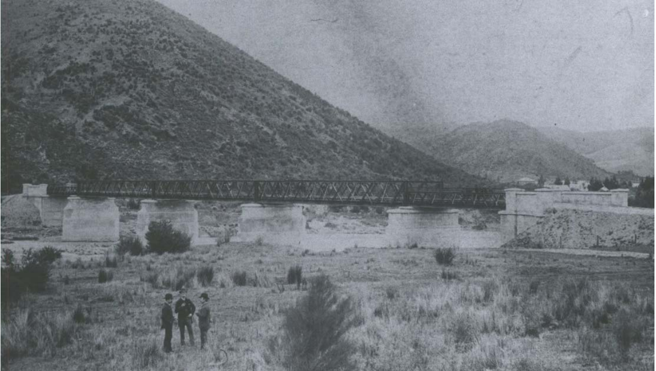
Figure 24: Beaumont Bridge in 1887 shortly after completion.
