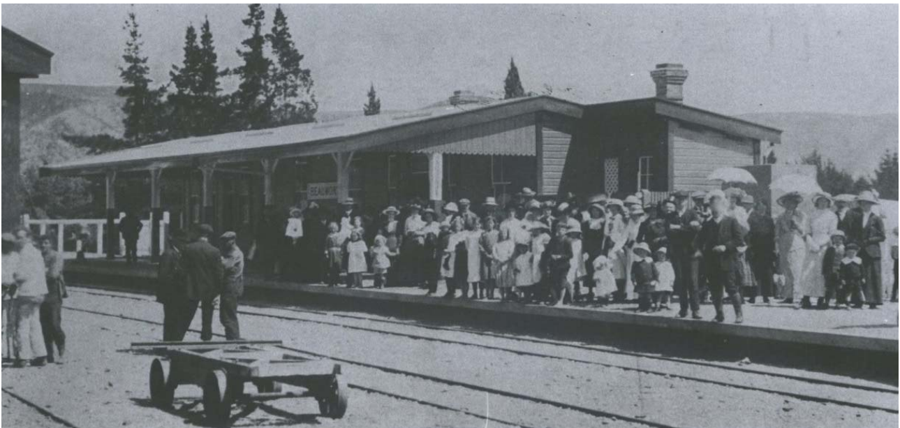
Figure 13: Beaumont Railway Station 1915.
