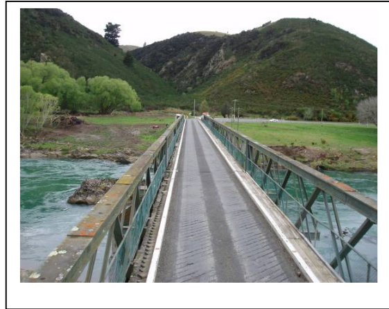
Looking towards Lawrence (East end of bridge)
