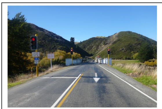
Traffic Signals to reduce dynamic load
