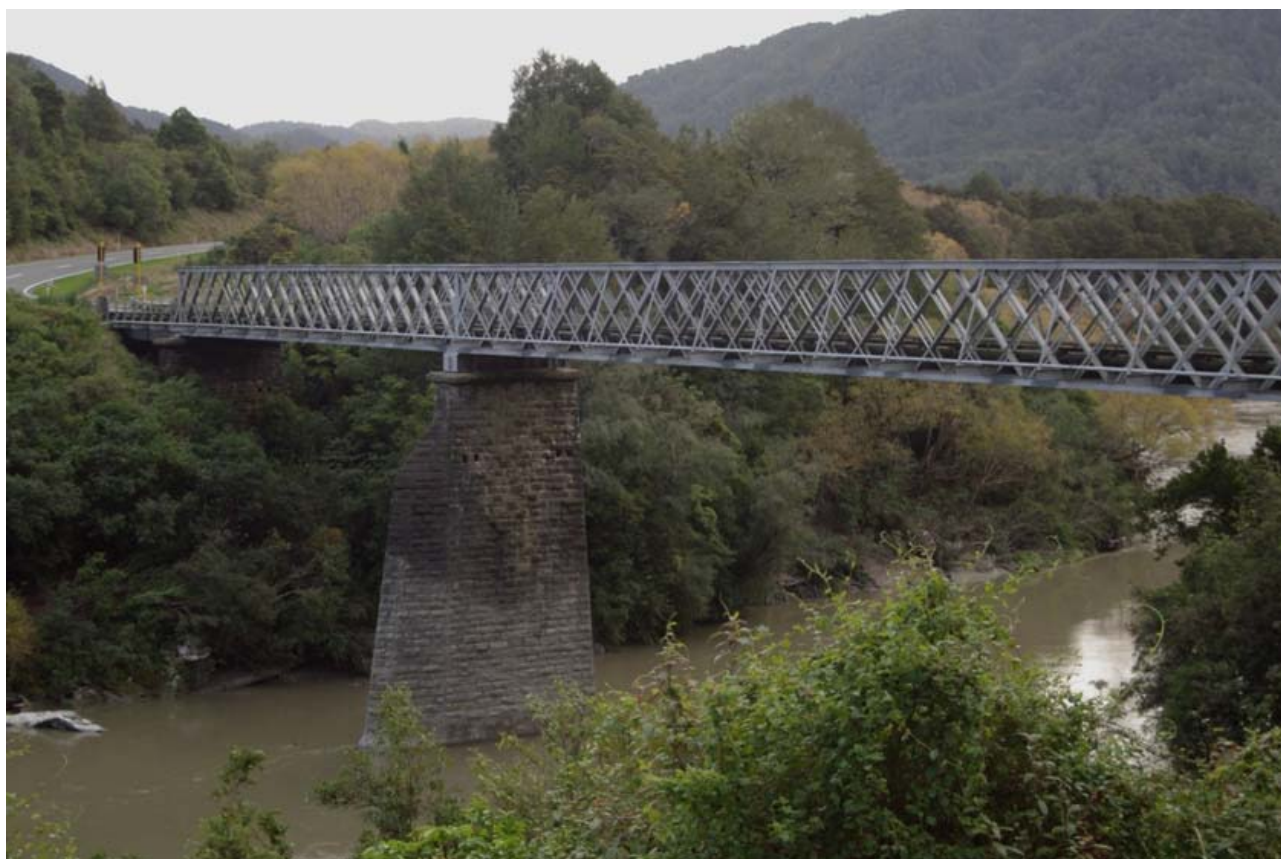
Figure 43: Iron Bridge, Lyell.
