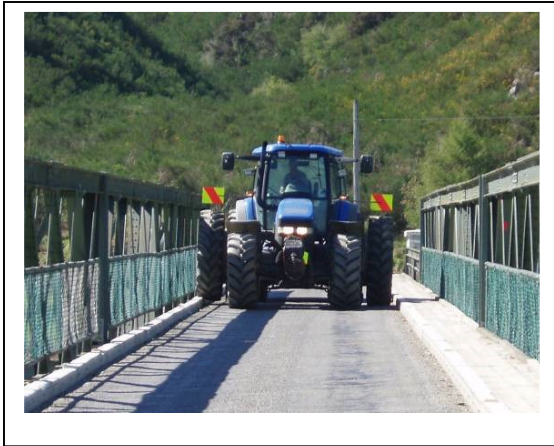
Single Lane shows the pedestrian walkway and timber kerb
