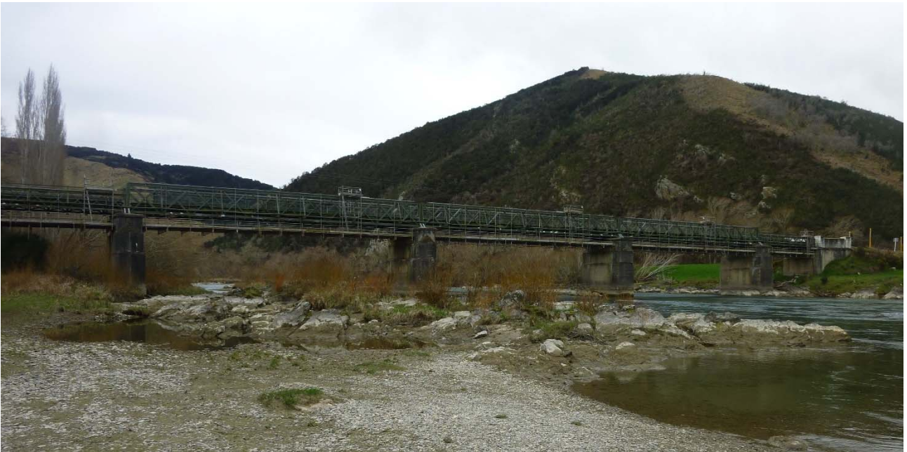
Figure 28: Beaumont Bridge viewed from south.
