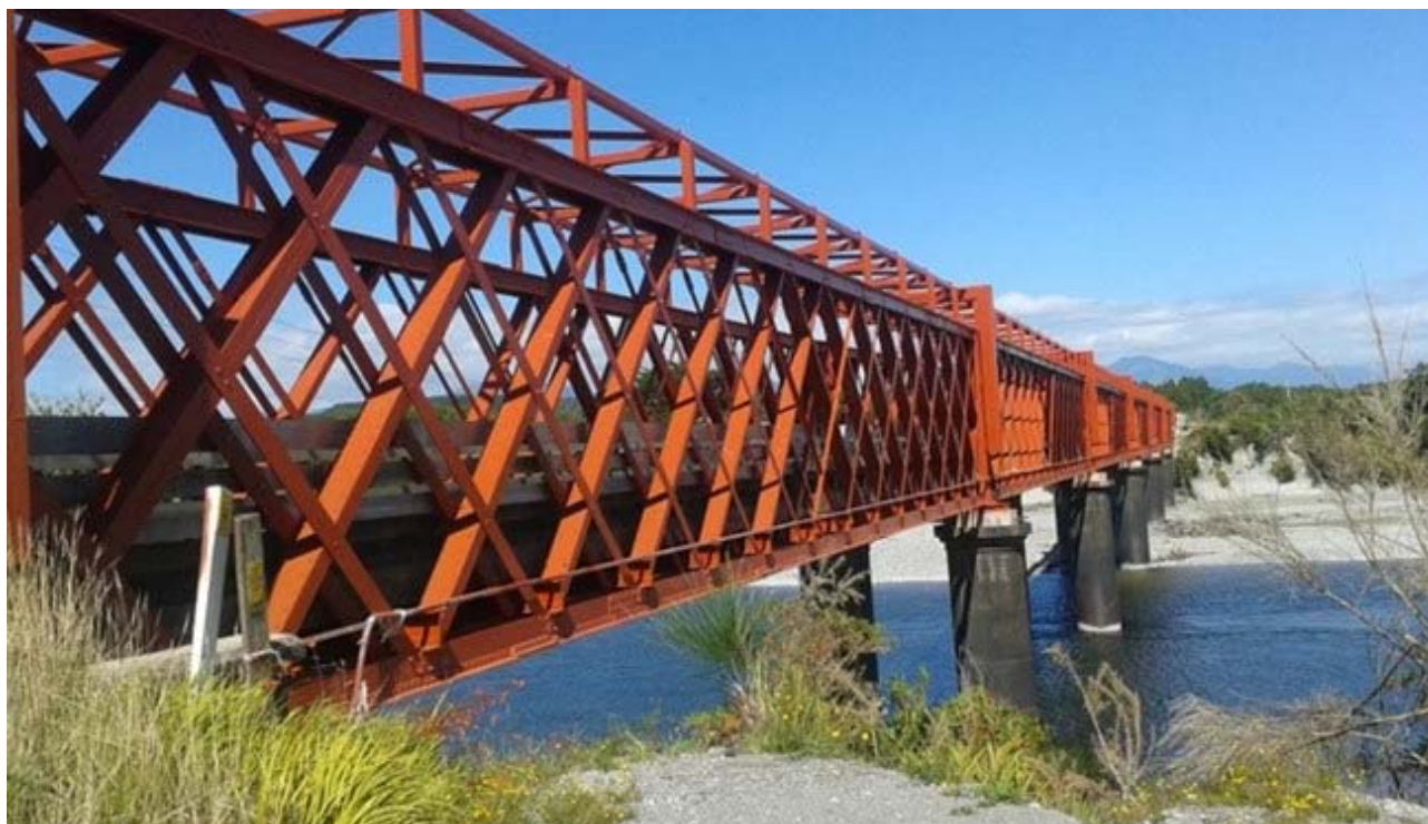
Figure 44: Taramakau Road and Rail Bridge, SH6.
