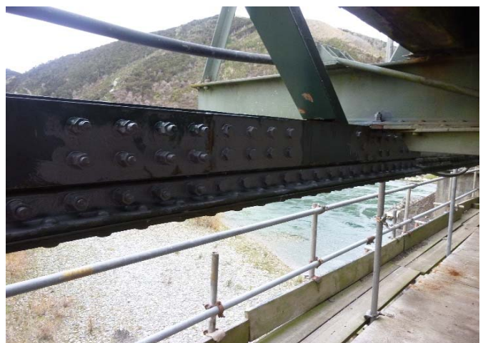
Figure 36: Recent repair of wrought iron bottom chord.
