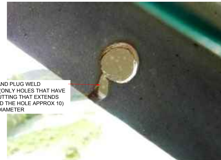
GAS CUT TIES - PLUG WELD
