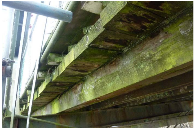
Figure 38: Timber bearers and edge of timber decking.
