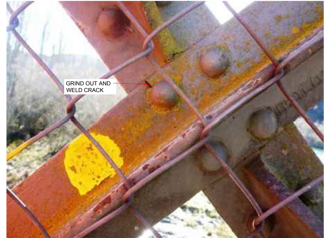
GAS CUT TIES - PLUG WELD
