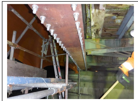
Additional Plate on the bottom chord strengthening.
