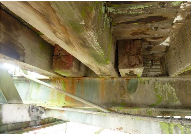
Figure 37: Timber bearers on wrought iron transom.
