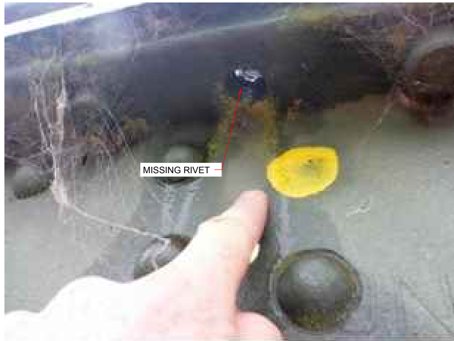
A RIVET IS MISSING ON THE TOP OF THE TOP CHORD, A M20 BOLT SHALL BE INSTALLED TO REPLACE THE MISSING RIVET. TOTAL PLATE THICKNESS IS 51mm
