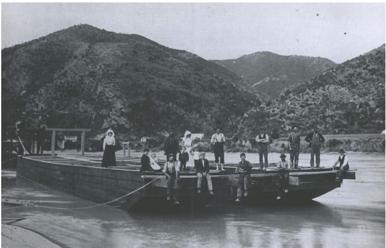
Figure 12: Pontoons of the Golden Gravel Dredging Co at their launching at Beaumont, c.1900.
