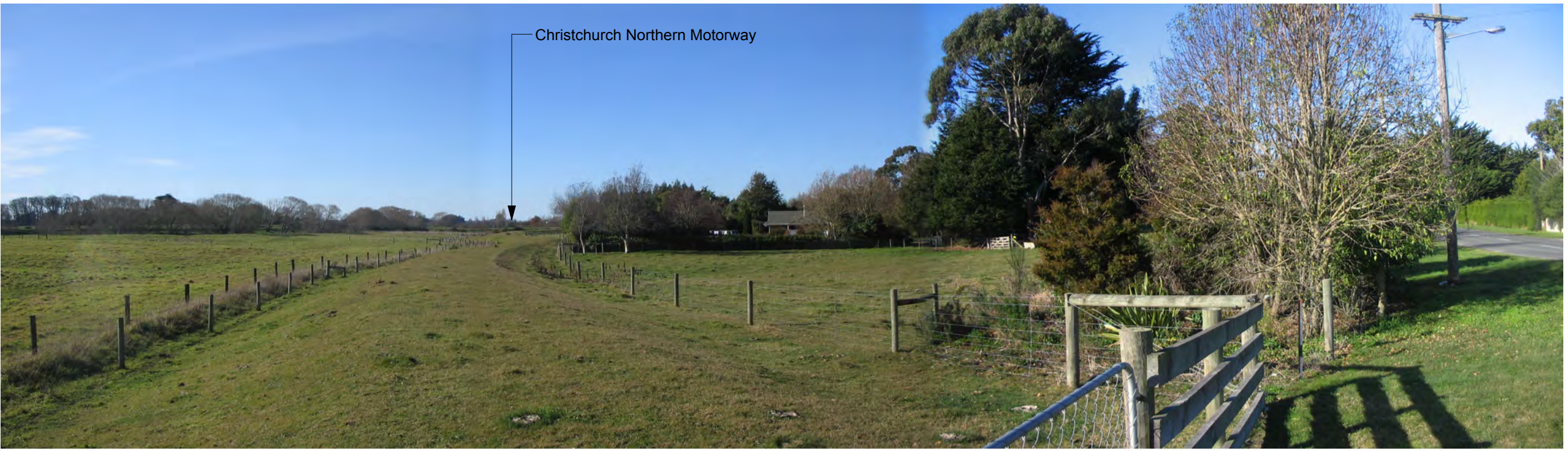
Photograph 4. As Built Christchurch Northern Motorway: Looking at Christchurch Northern Motorway at grade, approximately 700 metres away
