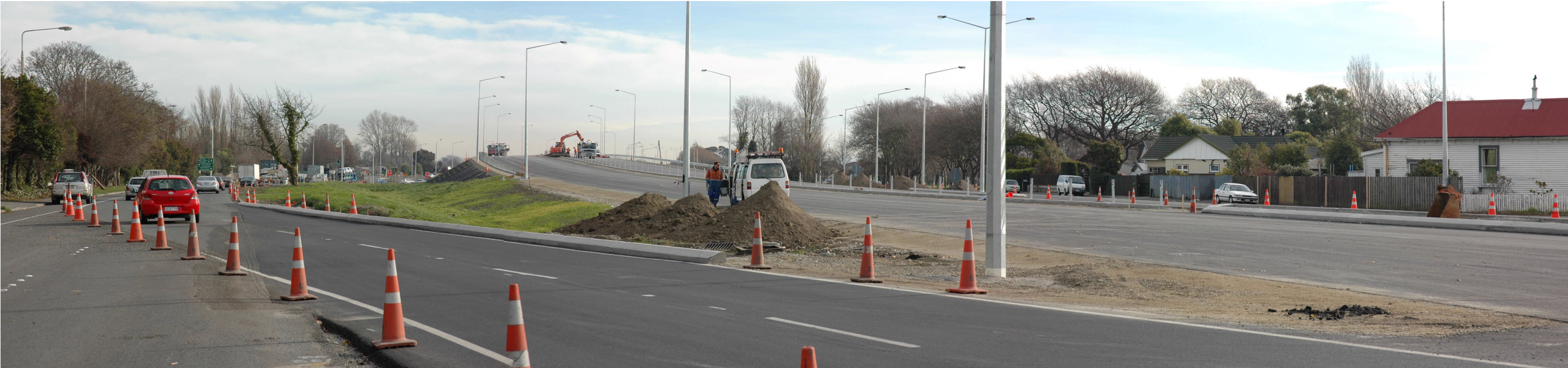
Photograph 5. CSM1 Brougham Street overbridge (Barrington Street) looking west
