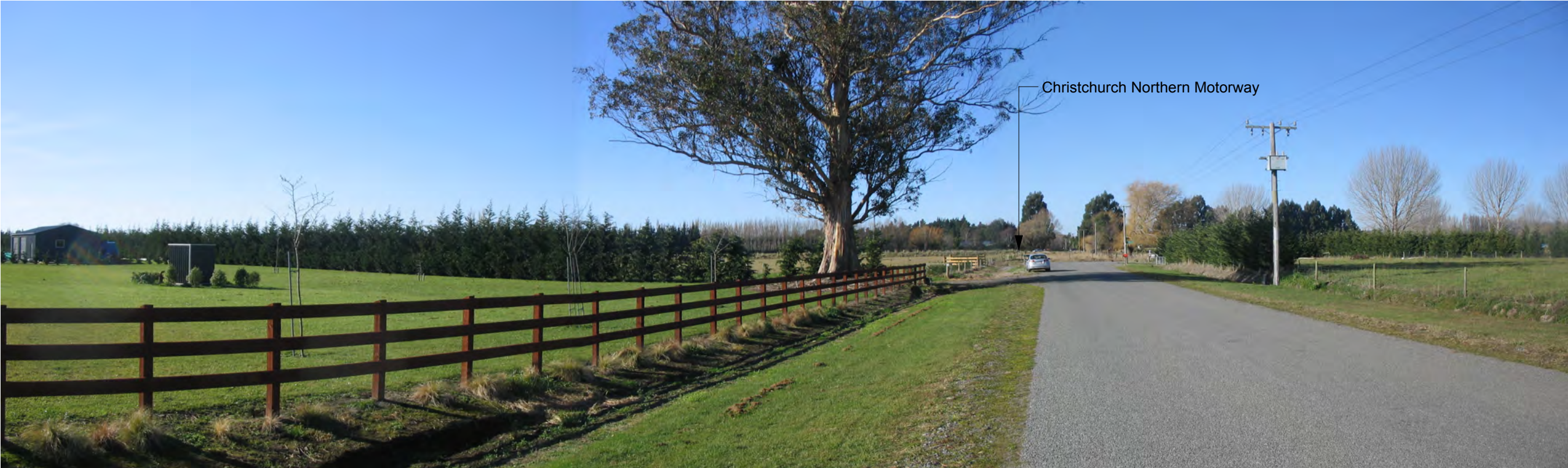
Photograph 2. As Built Christchurch Northern Motorway: Looking at Christchurch Northern Motorway at grade, approximately 280 metres away
