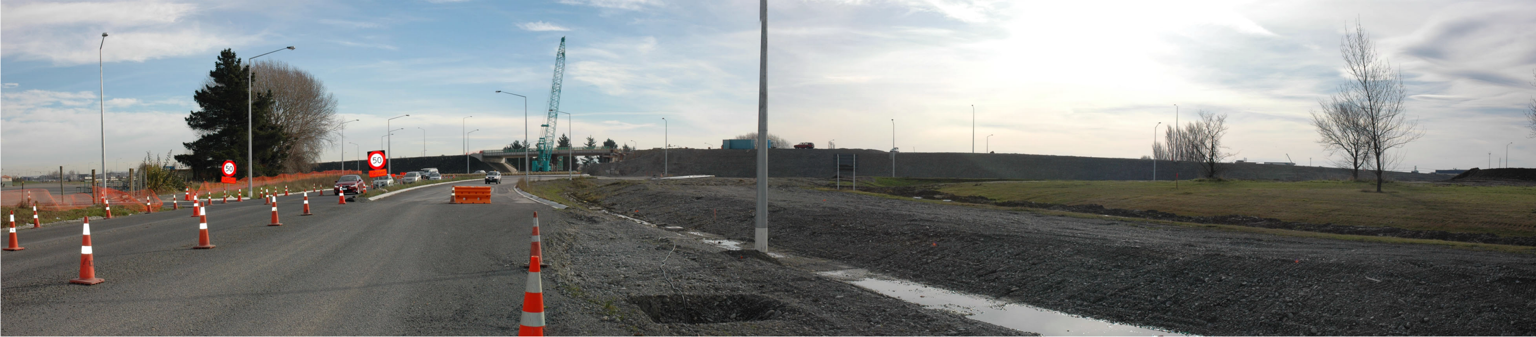
Photograph 6. CSM1 looking north to overbridge from Curletts Road
