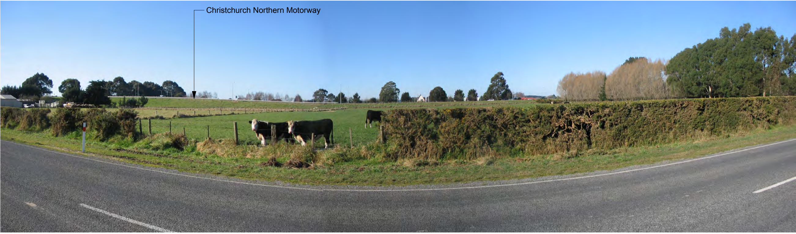
Photograph 3. As Built Christchurch Northern Motorway: Looking at an overpass on Christchurch Northern Motorway across relatively open land, approximately 200 metres away
