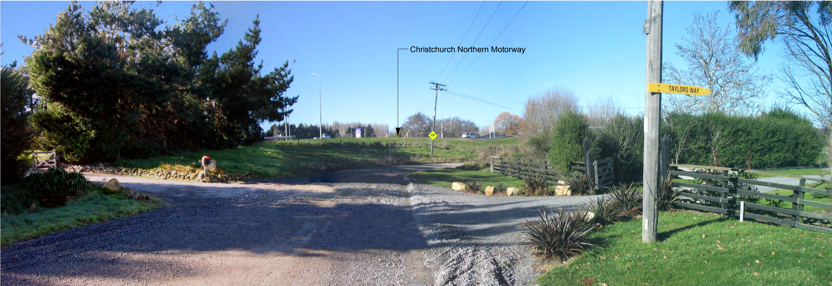
Photograph 1. As Built Christchurch Northern Motorway: Looking at an overpass on Christchurch Northern Motorway from a low elevation approximately, 100 metres away
