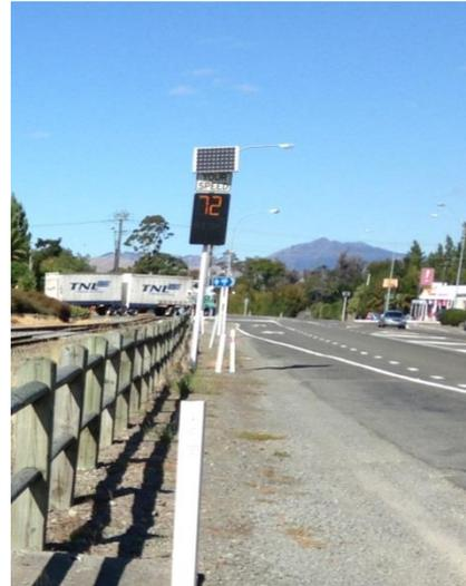
Figure 15-16: Solar speed sign
