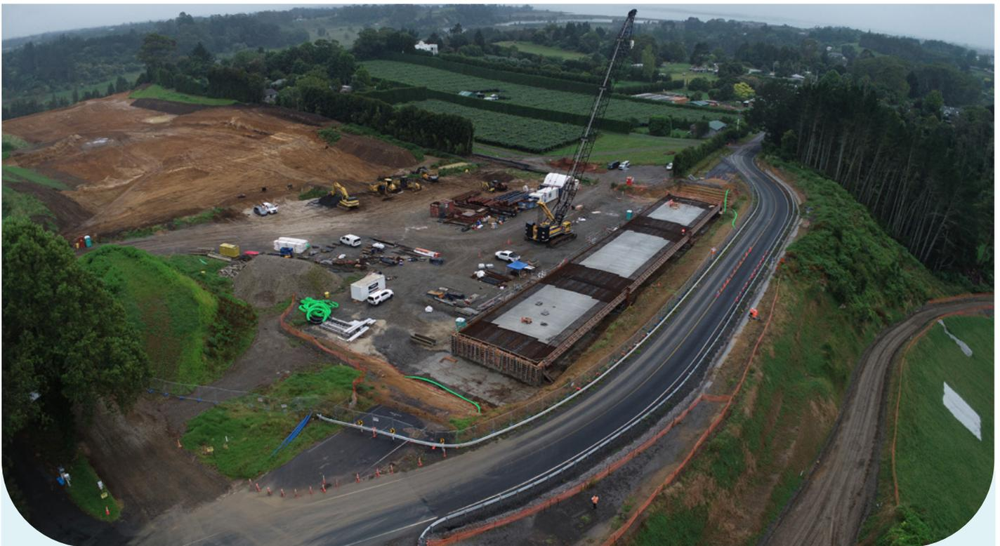
**Wairoa Road Overbridge:** Construction continues with utilities being realigned within the bridge structure, which is now due to complete early 2024. In the background we are removing approximately 660,000m<sup>3</sup> of material to get down to the finished road level.
