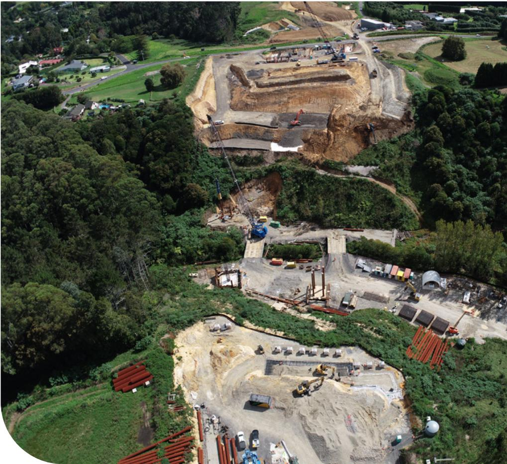
**Te Rangi Tuanehe (Minden Gully):** Temporary bridges have been created over the Hakao Stream allowing a one-way system across the stream for construction vehicles only. The construction vehicles go in via the left-hand bridge and out via the right-hand bridge.
