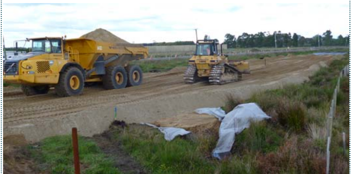
Parton Road temporary diversion underway
