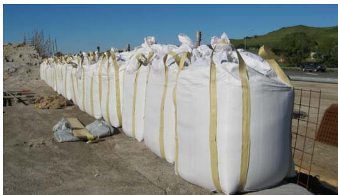
The first of 600 sand filled bags on the Mangatawa interchange
