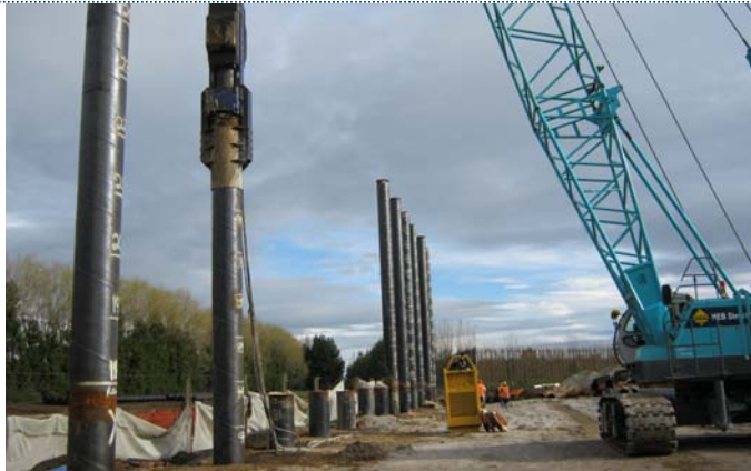
One of 16 piles being driven for the ECMT bridge
