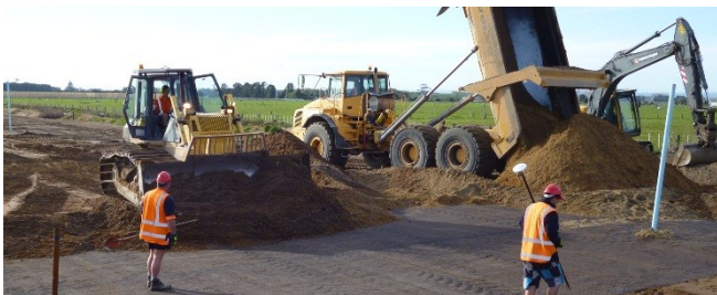
Above: Laying of geogrid material for strength.
