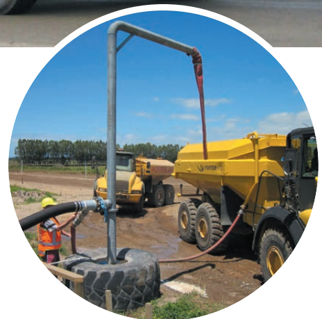
Water truck fill station - water is taken from a lined pond
