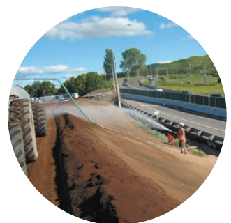
A dust suppressant is sprayed on to exposed dirt and sand, as it dries it forms a crust
