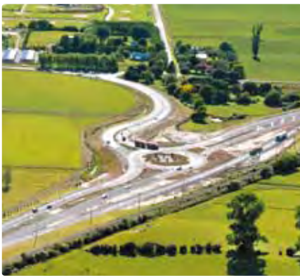
SH2/Domain Road roundabout - January 2011
