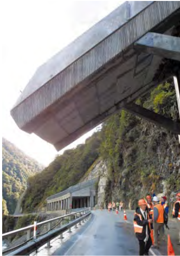
Waterfall chute with rock shelter in the background at Candy's Bend to Starvation Point on SH73.
