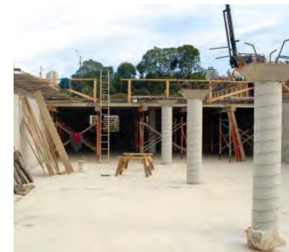
Treatment tank at Grafton Gully under construction.
