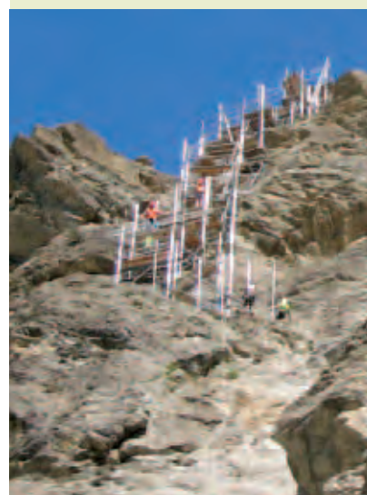
After: scaffolding on the Nevis Bluff enabled work to be carried out to stabilise the rock face.
