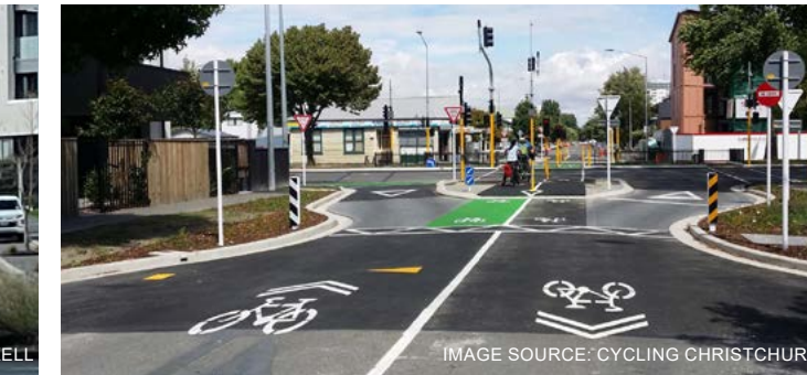
RAPANUI CYCLEWAY AT FITZGERALD AVENUE, CHRISTCHURCH
