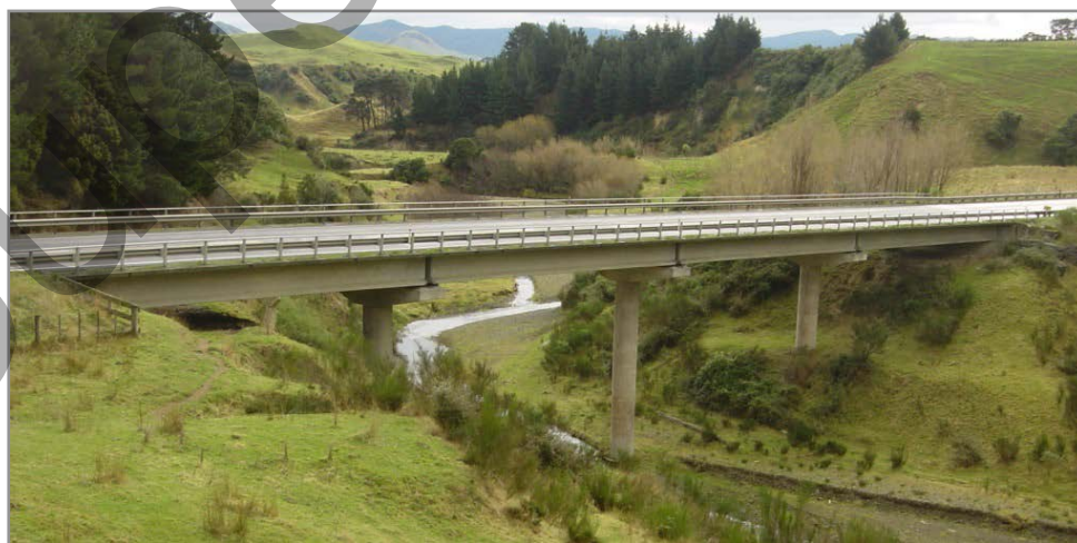
Figure C5B.1: Mangatewai-iti River Bridge looking to north
